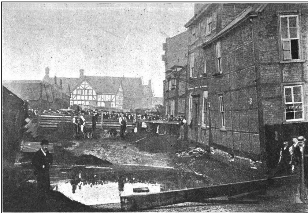
SUBSIDENCE NEAR THE DANE BRIDGE, NORTHWICH
