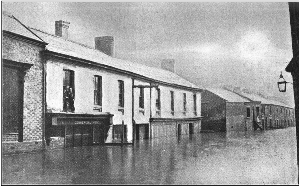
THIS ROAD WAS RAISED TWENTY FEET IN TWENTY YEARS. NONE OF THESE BUILDINGS IS NOW STANDING
