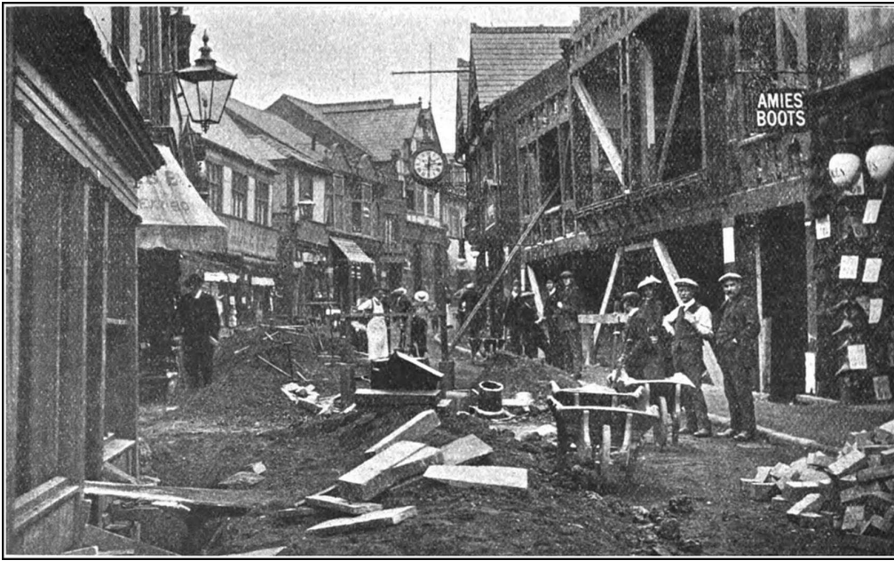
STREET-RAISING IN PROGRESS—HIGH STREET, NORTHWICH
