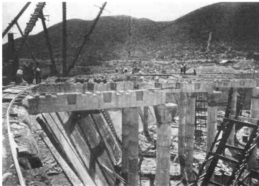
PLATE IX, FIG. 2.—SETTING PRIMARY BEAMS, SOUTH RESERVOIR.
