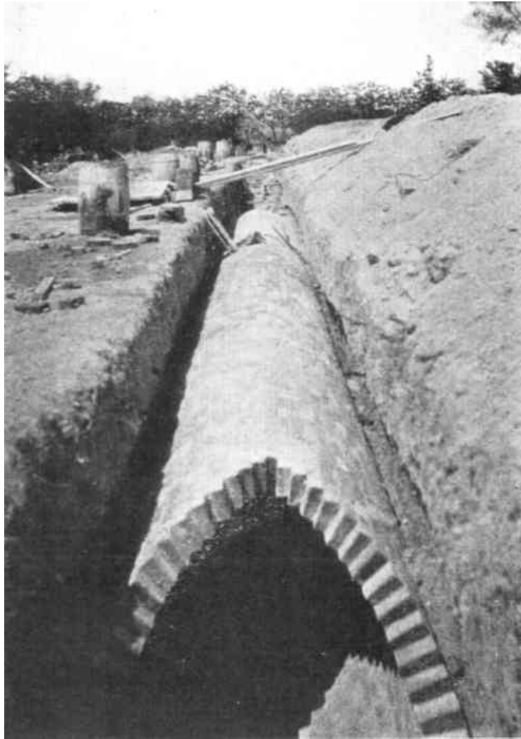
PLATE XXI, FIG. 1.—VIEW OF ARCH, OUTFALL SEWER.
