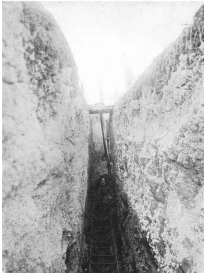
PLATE X, FIG. 2.—SETTING FORMS FOR SAN GERONIMO CULVERT.
