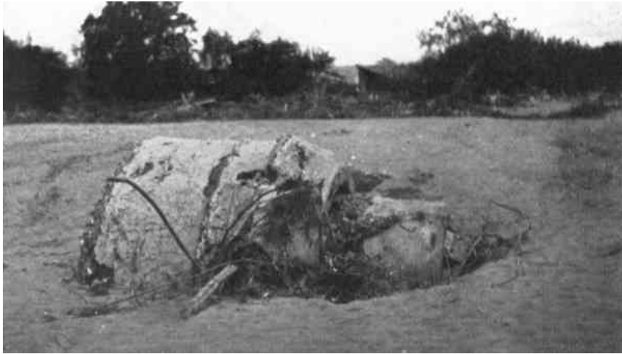
PLATE XXXI, FIG. 1.—FLUSH-TANK CARRIED DOWN BY FLOOD OF AUGUST 27TH-28TH, 1909.
