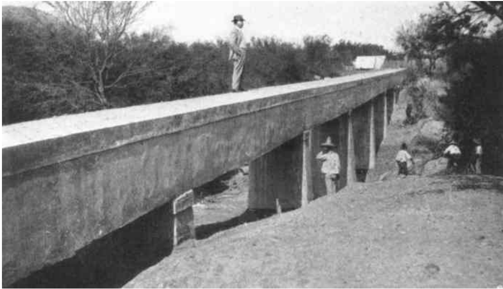
PLATE XXIII, FIG. 2.—VIEW OF ESTANSCIA BRIDGE, COMPLETED.
