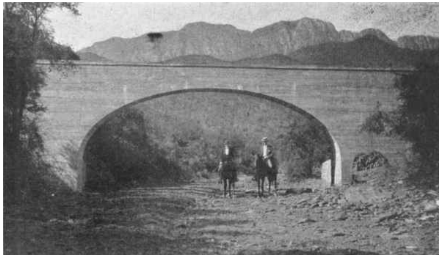
PLATE IV, FIG. 2.—ELLIPTICAL ARCH BRIDGE CARRYING ESTANZUELA AQUEDUCT.
