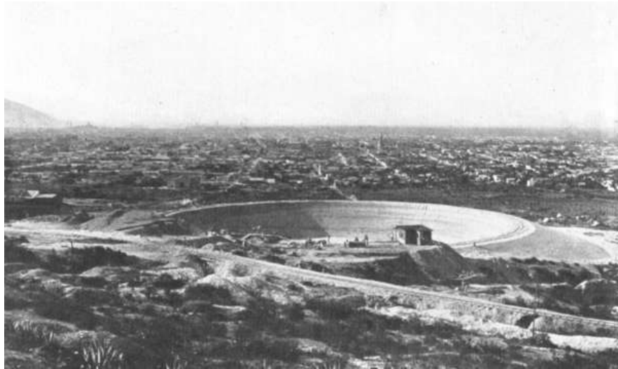
PLATE VIII, FIG. 1.—GENERAL VIEW OF EXCAVATION AND EMBANKMENT FOR SOUTH RESERVOIR BEFORE LINING.
