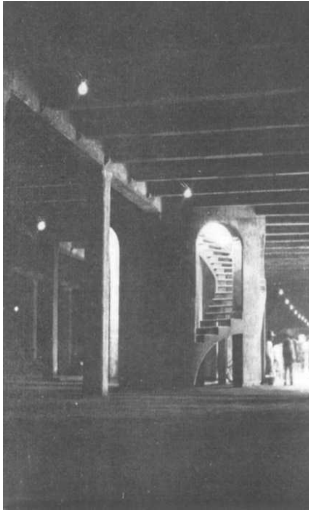
PLATE XVII, FIG. 2.—CENTRAL TOWER AND STAIRWAY, OBISPADO RESERVOIR.
