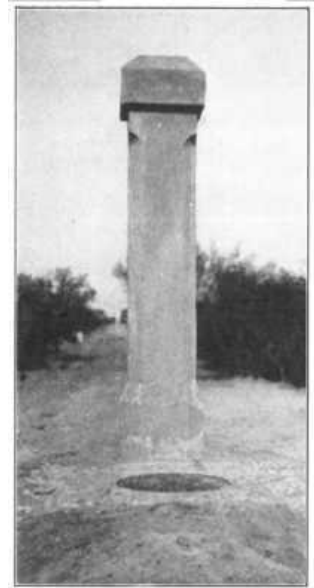
PLATE XXI, FIG. 2.— VENTILATING COLUMN AND MANHOLE, OUTFALL SEWER.
