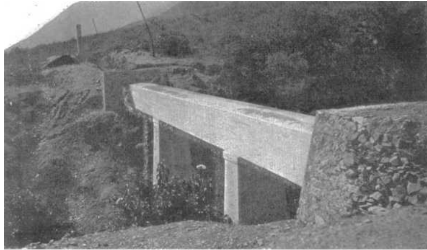
PLATE IV, FIG. 1.—TYPICAL REINFORCED CONCRETE GIRDER BRIDGE, ESTANZUELA AQUEDUCT.
