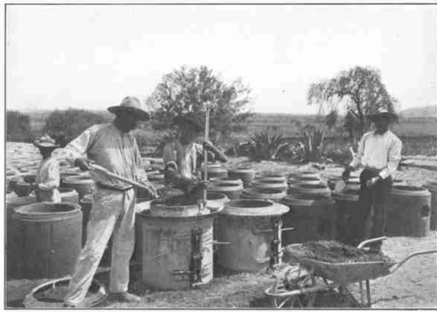
PLATE III, FIG. 2.—STEEL FORMS FOR MOULDING CONCRETE TUBES, ESTANZUELA AQUEDUCT.
