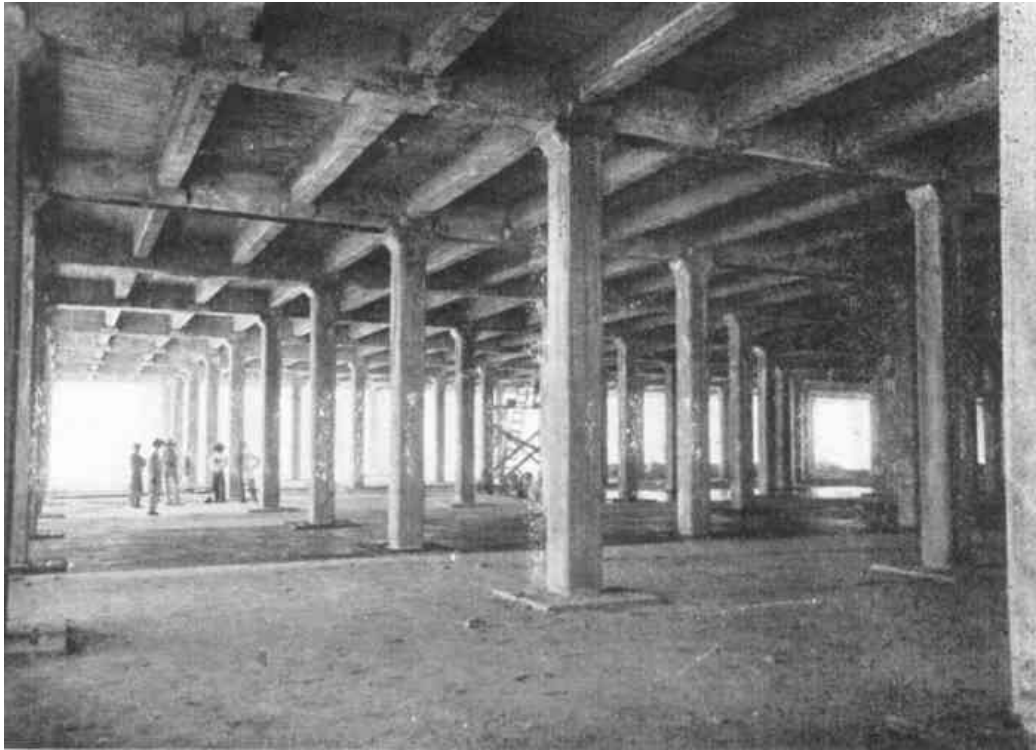
PLATE XVI, FIG. 1.—PREPARING FLOOR FOR CONCRETING, OBISPADO RESERVOIR.
