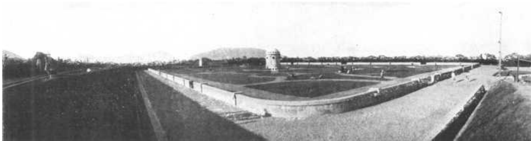
PLATE XVIII, FIG. 2.—VIEW OF ROOF OF OBISPADO RESERVOIR, LOOKING NORTH.
