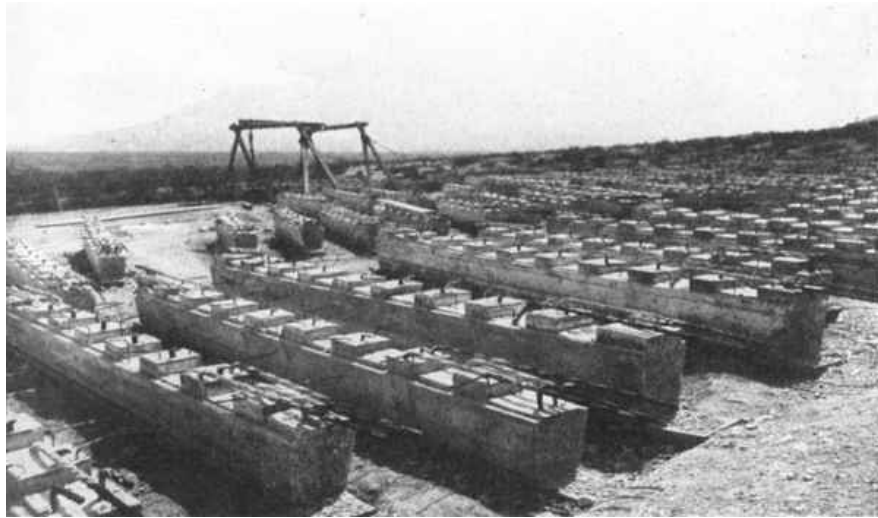
PLATE IX, FIG. 1.—VIEW OF SEPARATELY MOULDED SECONDARY BEAMS IN YARD BELOW SOUTH RESERVOIR.
