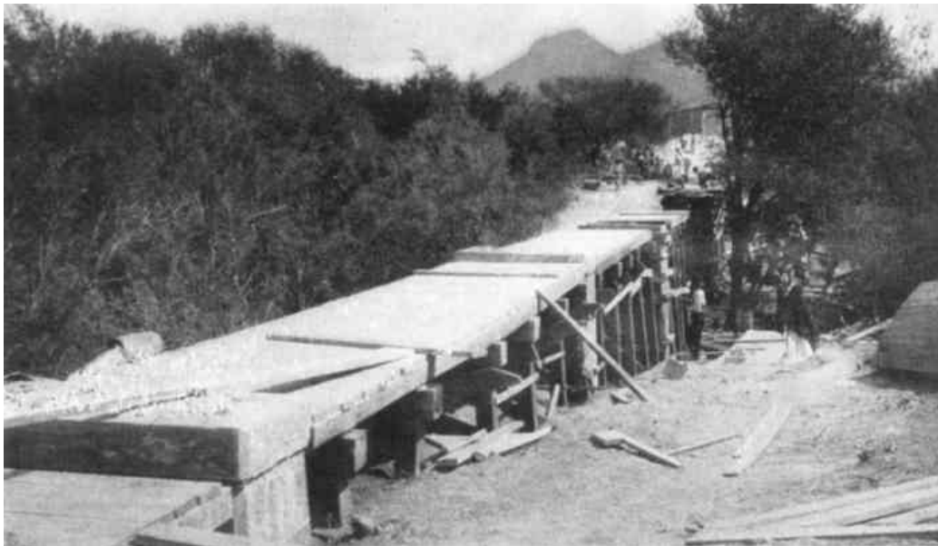
PLATE XXIII, FIG. 1.—FORMS FOR MAIN GIRDETS, ESTANCIA BRIDGE, OUTFALL SEWER.
