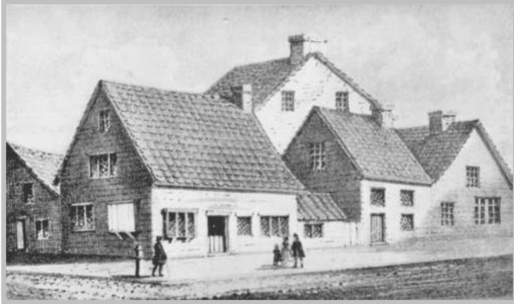
VIEW OF OLD BUILDINGS IN WILLIAM STREET, LOOKING TOWARDS MAIDEN LANE, 1800.
