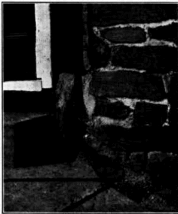
FIGURE 19.—Defects in foundations, such as the opening to the right of the step, are often the cause of rat infestation in old buildings
