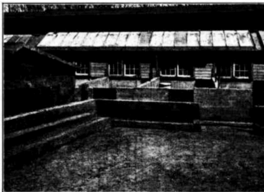
FIGURE 11.—Rat proof pigpens and feeding troughs are easy to keep clean and sanitary, and rats have little opportunity to steal the feed
