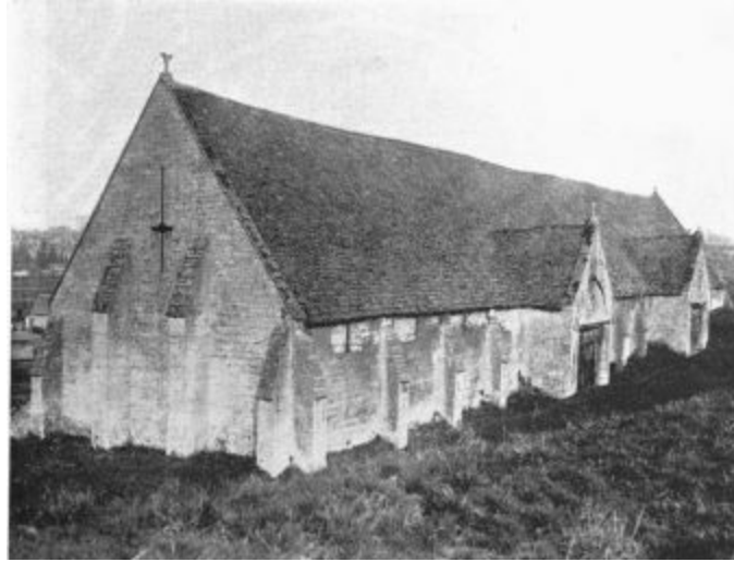
FIG. 43. Fourteenth century barn, Barton Farm, Bradford-on-Avon, Wiltshire. From the South-West. The barn exhibits numerous Gothic features of the period; angle buttresses, transept-like porches, gable crosses, &c. The windows, of which those at the ends are cruciform, are narrow slits, with wide splays internally. The Glastonbury barn is one of the finest in the country; the parochial tithe-barn was a much smaller building.
