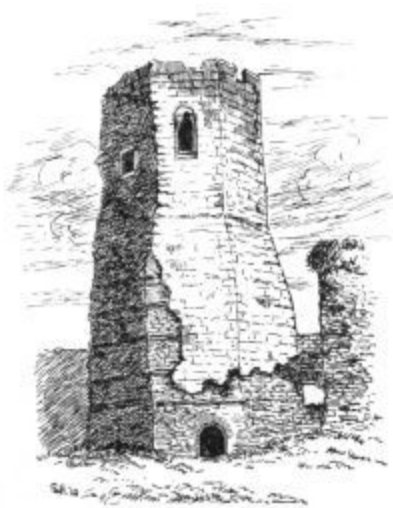
FIG. 5. The “pharos” or lighthouse, near the church within Dover Castle (Bloxam’s Gothic Eccles. Architect. ). The building is hexagonal externally, and square within. The lower part is composed of flints and rubble, with bonding courses of Roman tiles. The upper part of the tower belongs to the Tudor period. The doorway shown in the drawing has now been blocked up.
