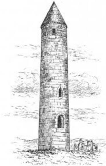
FIG. 28. Round tower of Devenish, on Devenish Isle, Lower Lough Erne, near Enniskillen. Height, 84 feet; doorway, 9 feet from the ground; walls, 4 feet thick. The windows approximately face the Cardinal Points. A string course will be seen around the base of the conical cap.
