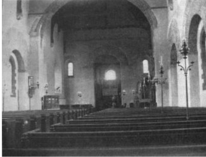
FIG. 3. Interior of Brixworth Church, Northampton. Chancel and eastern portion of nave. The Saxon arches are constructed of hard red Roman bricks or tiles, set edgewise. The arches spring from square, massive piers which have simple abaci. The materials were evidently obtained from some edifice previously in existence near the site of the church.
