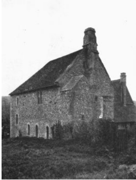
FIG. 46. Clergy, or Parsonage house, West Dean, Sussex (c. A.D. 1280). View from North end. The building, which is of stone, consists of a hall (30 ft \times 15 ft internal measurement), with a story above. The walls are 2 ft 6 in. in thickness. The solar, or loft, is approached by a stone newel staircase, built in the buttress-like projection, which is seen at the North-East angle. The chimney is elaborately constructed. In the east wall a double-lighted window, with trefoiled heads, is visible. (For fuller description, see Vict. Hist. of Sussex , II. p. 383; A. Hussey, Churches of Kent, Sussex, and Surrey , 1852, p. 219; Sussex Archaeol. Coll. III. pp. 13-22.)
