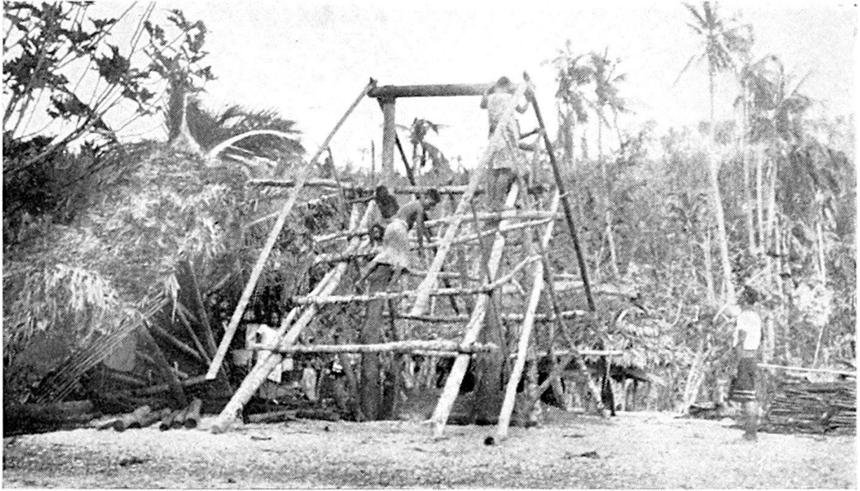
Rebuilding the village after a hurricane
