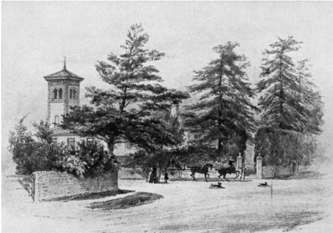
HARTING GRANGE. SOUTH ENTRANCE.
