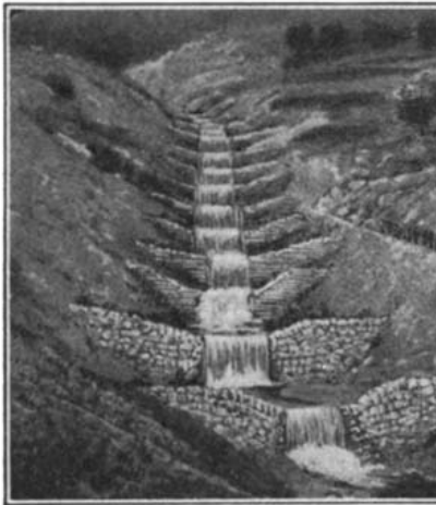
Working to prevent erosion after the removal of the forest in the French Alps.
