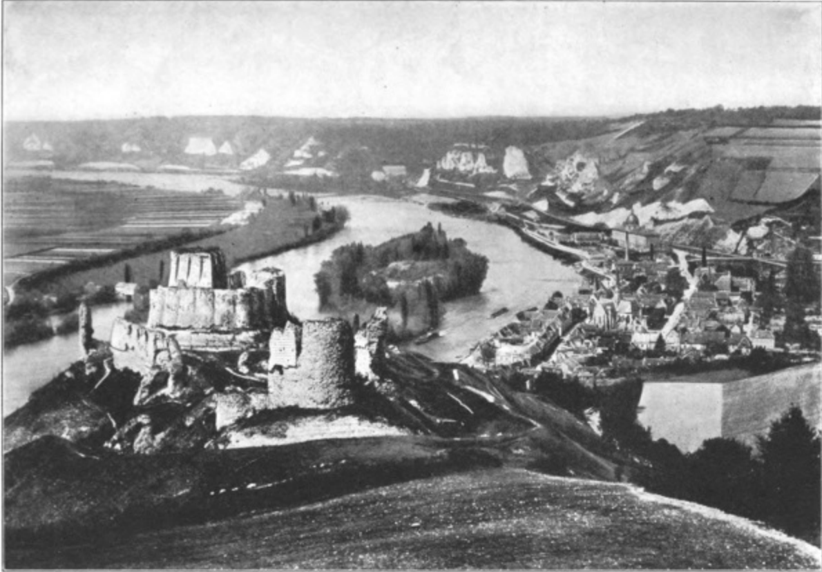
LE PETIT ANDELY: VIEW OF THE TOWN AND CHÂTEAU GAILLARD
