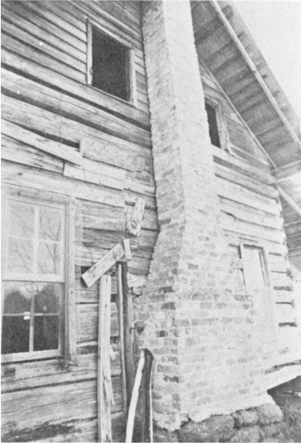
17. Loft windows. Wiley McNeill house, Clarke County. ca. 1820-30.
