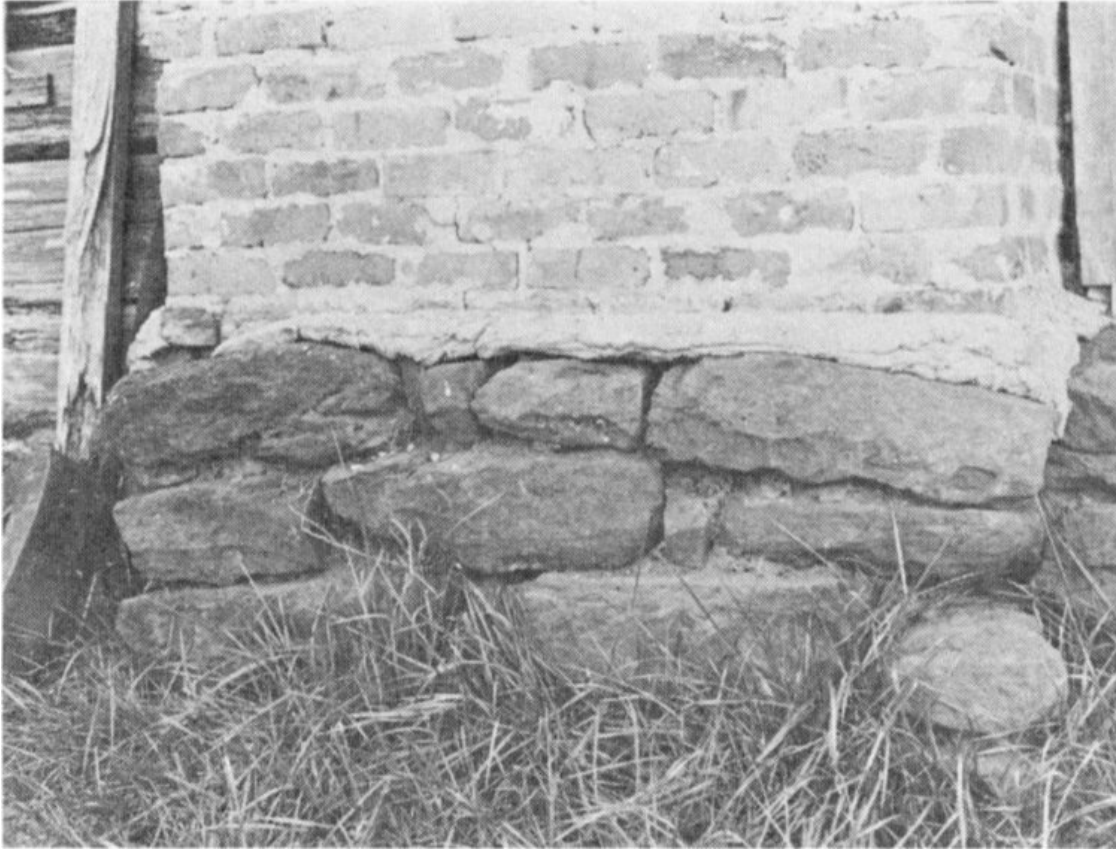
16. Bricks replaced mud-and-stick chimney in 1951. The original foundation stones remain. Wiley McNeill house, Clarke County.
