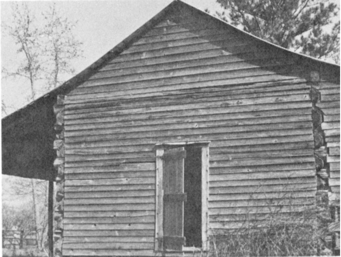
19. Window shutter. John Walters cabin, Rankin County, 1860s. Present owner: James Huff
