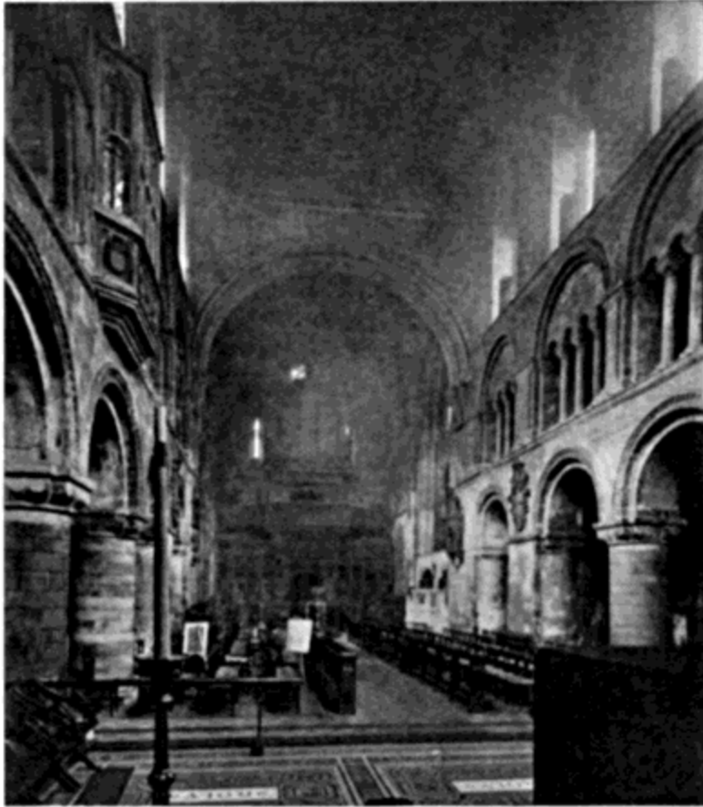
INTERIOR FROM THE EAST, SHOWING PRIOR BOLTON'S GALLERY
