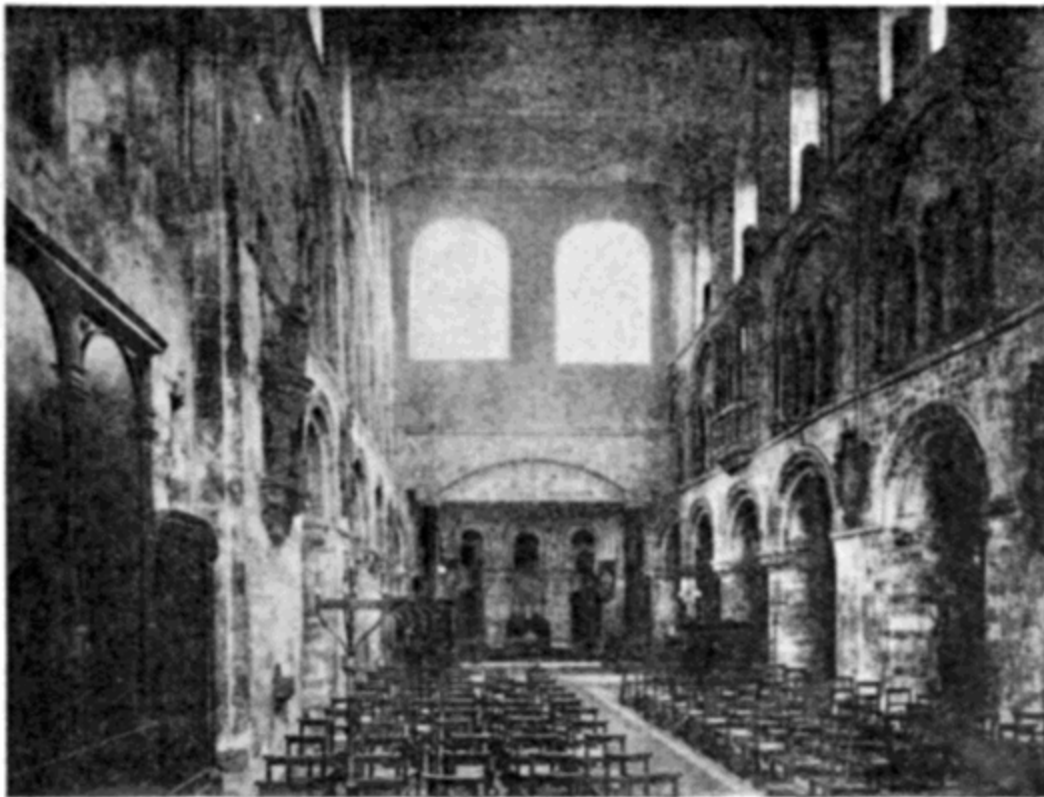
THE CHOIR BEFORE RESTORATION, SHOWING THE FACTORY FLOOR EXTENDING OVER THE APSE AND SUPPORTED BY TWO IRON COLUMNS
