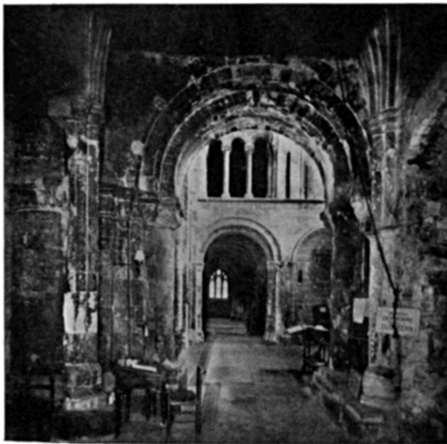
THE SOUTH AISLE FROM THE WEST, SHOWING THE EARLY ENGLISH SHAFTS
