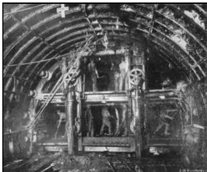
DRIVING THE TUNNEL FOR THE WATERLOO AND CITY RAILWAY.
