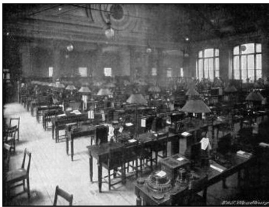
A PORTION OF A TELEGRAPHIC OPERATING ROOM AT THE GENERAL POST OFFICE, LONDON.
