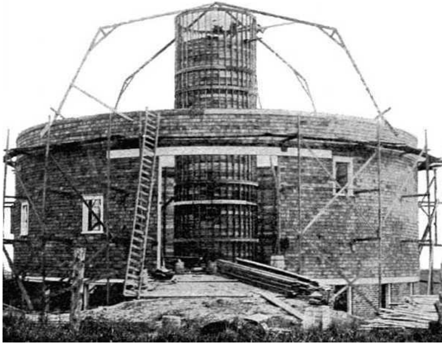
FIG. 14. SHOWING HEIGHT AND CONSTRUCTION OF SILO, SIDING COMPLETED, AND FOUR MAIN RAFTERS IN PLACE.
