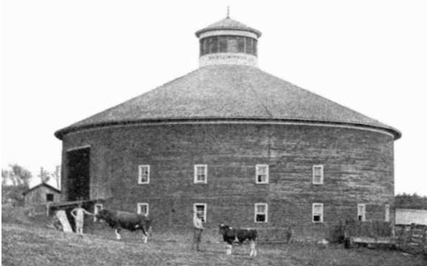
FIG. 34. BARN 92 FEET IN DIAMETER; TWO ROWS OF COWS HEADED TOGETHER; SILO IN CENTER.
