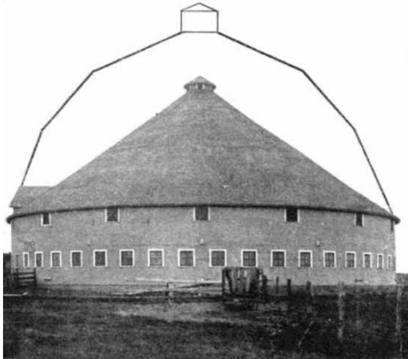
FIG. 1. BARN NO. 5. 100 FEET IN DIAMETER, SCALE 20 FEET TO ONE INCH; SHOWING INCREASED MOW CAPACITY GIVEN BY SELF-SUPPORTING ROOF.
