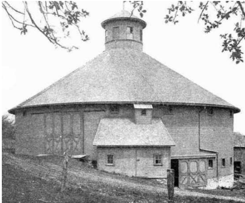
FIG. 26. BARN NO. 2. 80 FEET IN DIAMETER; ENGINE ROOM IN FOREGROUND.
