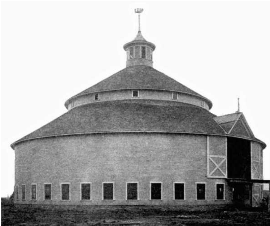
FIG. 30. BARN NO. 4. 90 FEET IN DIAMETER; ONE OF THE FEW DAIRY BARNs WITH SUFFICIENT LIGHT; SAME SCALE AS DRAWING ON PAGE 37 .
