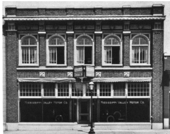
Face Brick Store Front, St. Louis, Mo. Preston J. Bradshaw, Architect
