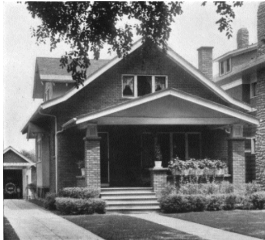
Attractive Small Face Brick House, Buffalo, N. Y. Thos. A. Fisher, Designer
