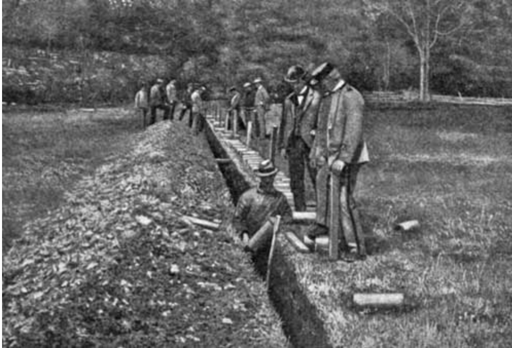
FIG. 9. LAYING A TILE DRAIN
