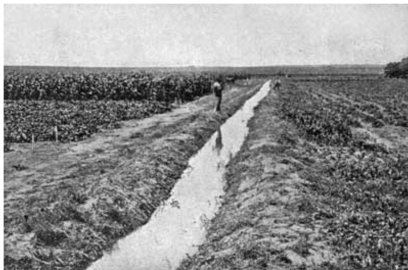
FIG. 287. THE MAIN DITCH OF AN IRRIGATION PLANT
