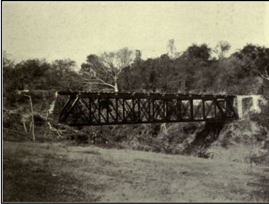
DECK BRIDGE ON SALVADOR RAILWAY.
