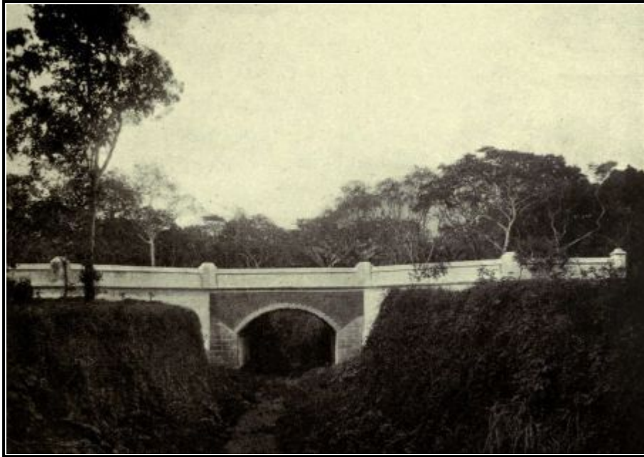
SIDE VIEW OF "EL ROTULO" BRIDGE.
