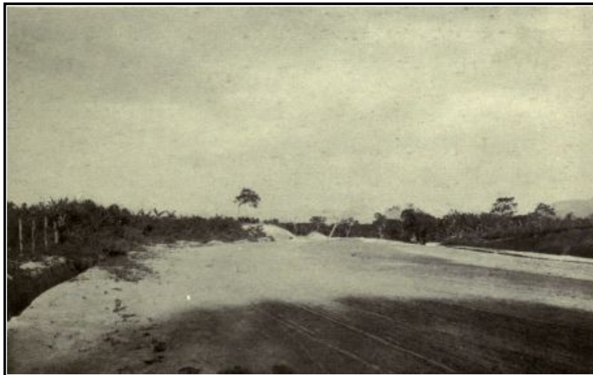
THE FAMOUS AVENIDA UNDER CONSTRUCTION.
