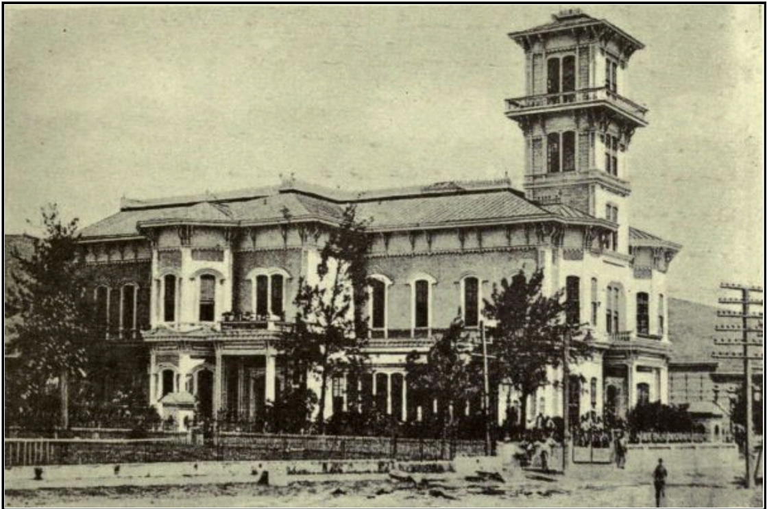
GOVERNMENT BUILDING ("CASA BLANCA"), SAN SALVADOR.
