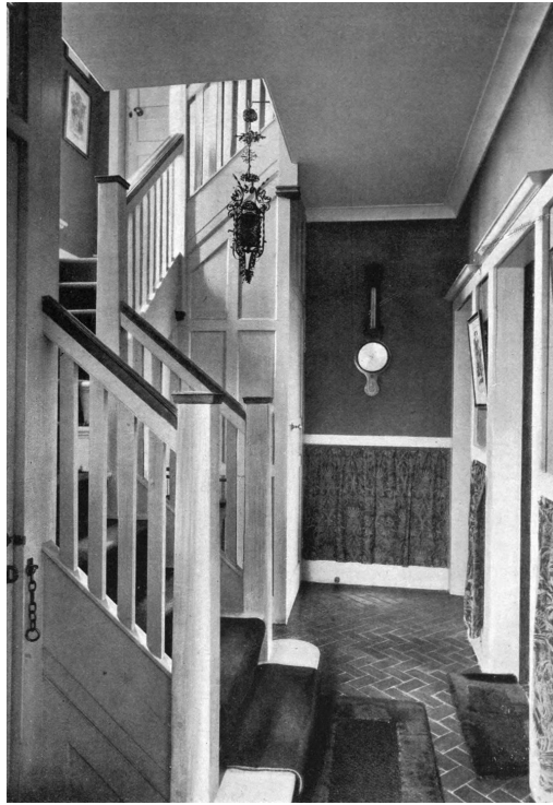
PLATE XLI. STAIRCASE OF SINGLE COTTAGE. SEE PAGE 44 .
