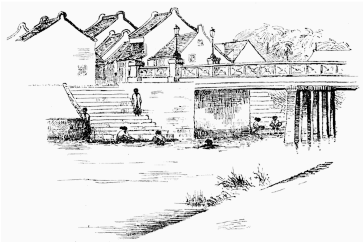
BRIDGE LEADING TO THE PAZER BAROE, BATAVIA.
