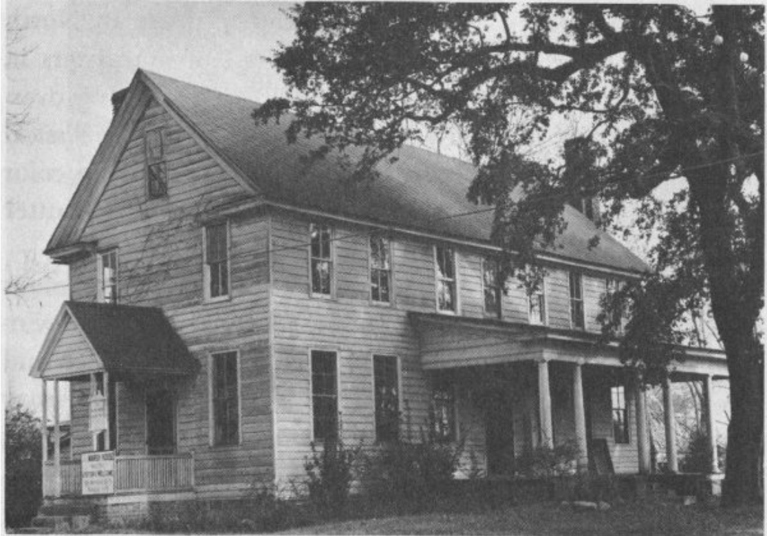
FIGURE 11. THE PALMER HOUSE BEFORE RESTORATION.
