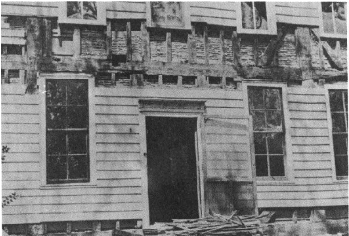
FIGURE 28. THE PALMER HOUSE, BATH, DURING RESTORATION.
