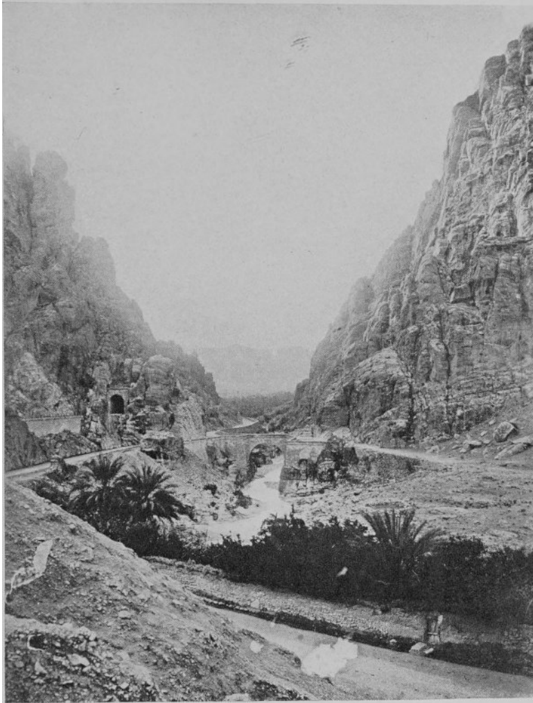
The Bridge of the Third Legion at El Kantara
