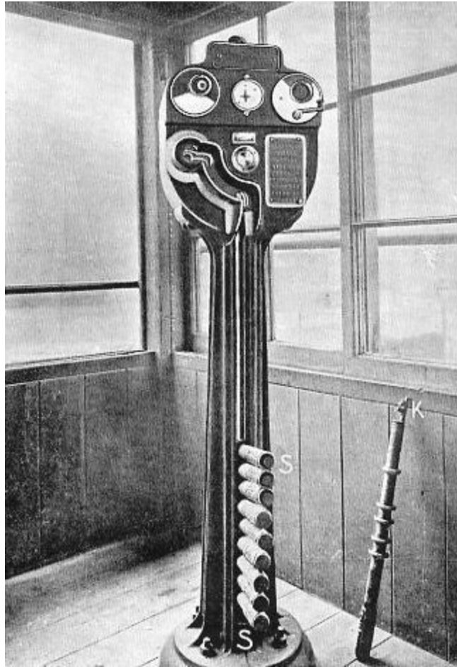
FIG. 101.—An electric train staff holder: s s, staffs in the slot of the instrument. Leaning against the side of the cabin is a staff showing the key \kappa at the end for unlocking a siding points between two stations. The engine driver cannot remove the staff until the points have been locked again.
