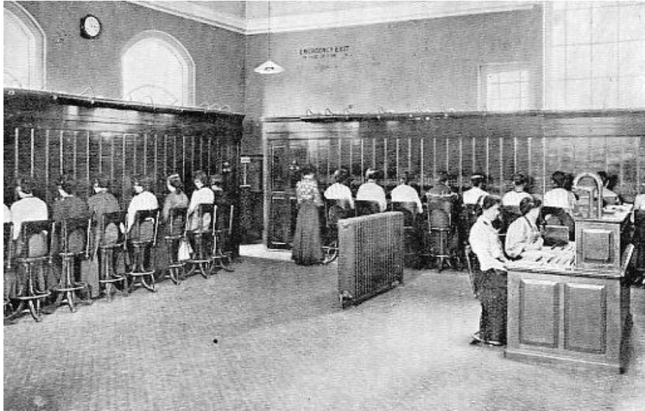
A TELEPHONE EXCHANGE.
