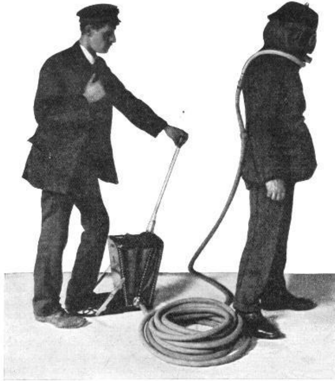
FIG. 36.—Smoke Helmet, Flexible Tubing, and Foot Bellows ( Siebe, Gorman & Co. )
