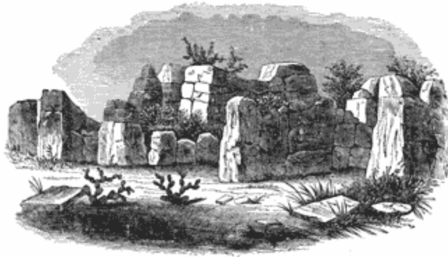
Fig. 57.—End View of Fortress Walls at Cuzco.
