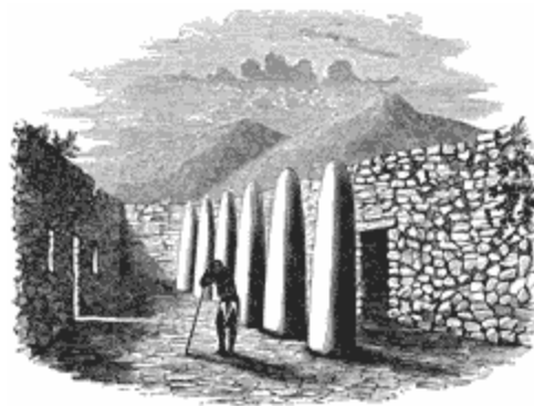
Fig. 31.—Great Hall at Mitla.
