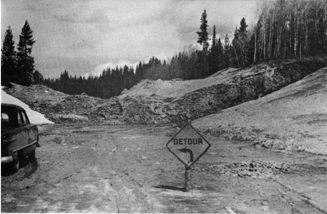
Figure 17. Slide blocking main highway in northern part of Grand Teton National Park. National Park Service photo by Eliot Davis, May 1952.
