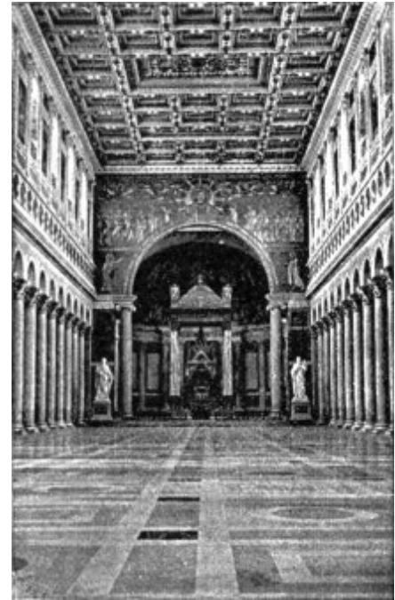
FIG. 68.—ST. PAUL BEYOND THE WALLS. INTERIOR.
