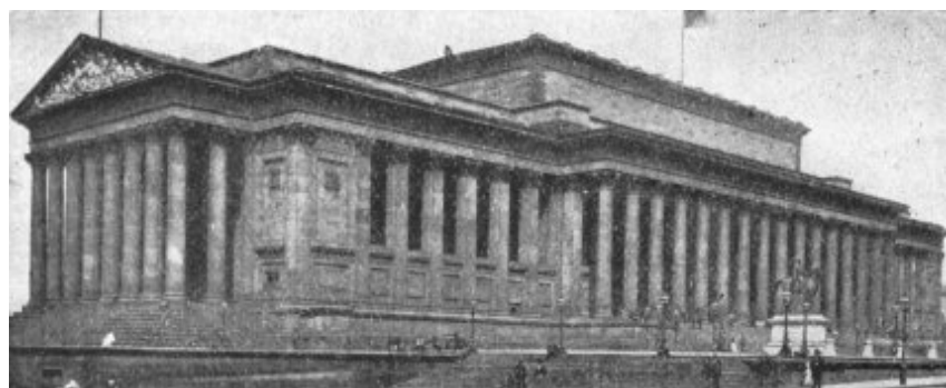
FIG. 199.—ST. GEORGE'S HALL, LIVERPOOL.
