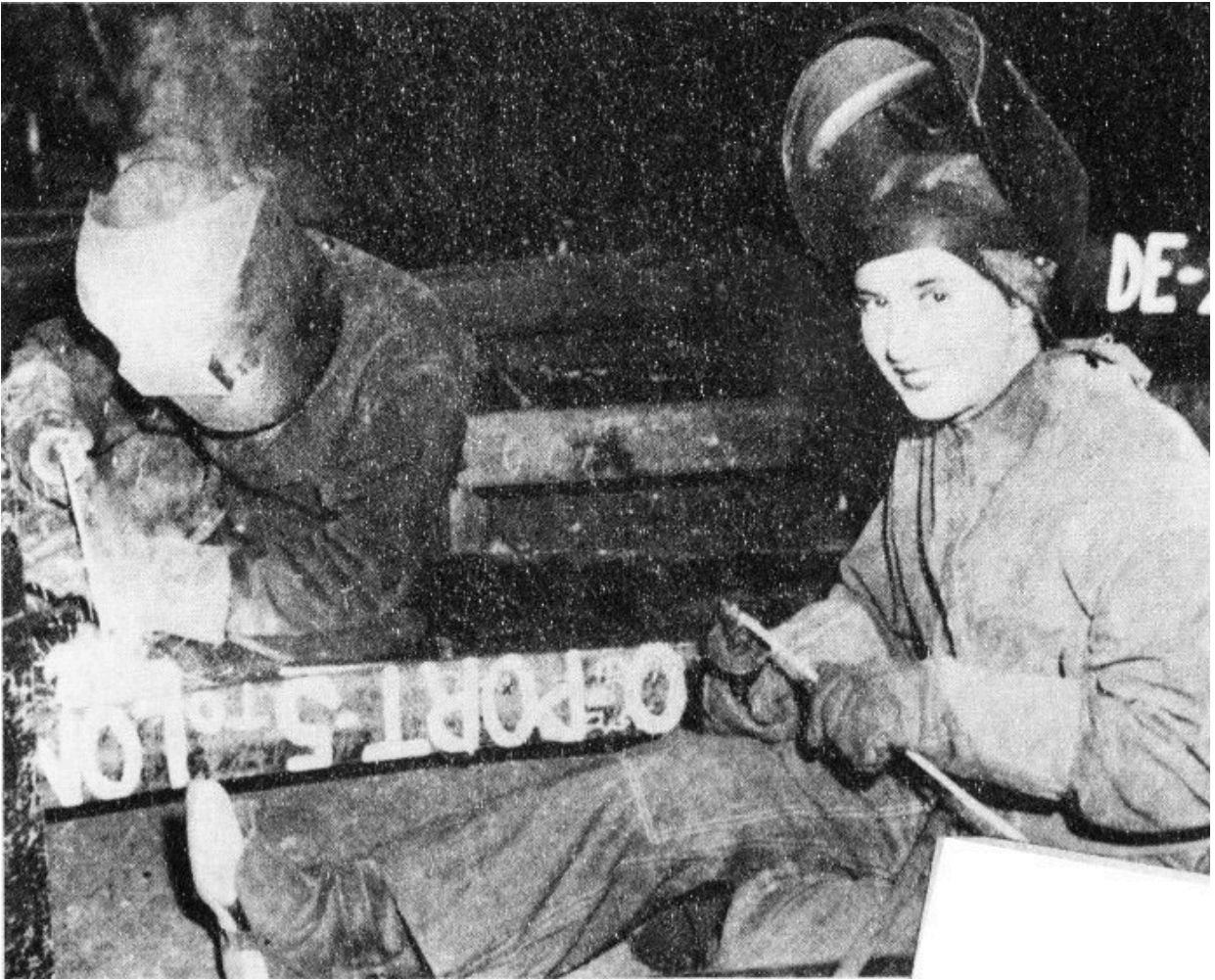
Welders at Charlestown during World War II.
