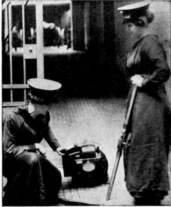
Reading the Gas Meter.
