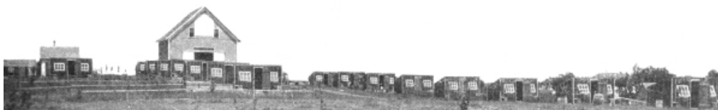
Colony chicken houses on farm of G. M. Gowell, of the Maine Agricultural Experiment Station, Orono, Maine. The roofs are covered with PAROID, sides with NEPONSET.
