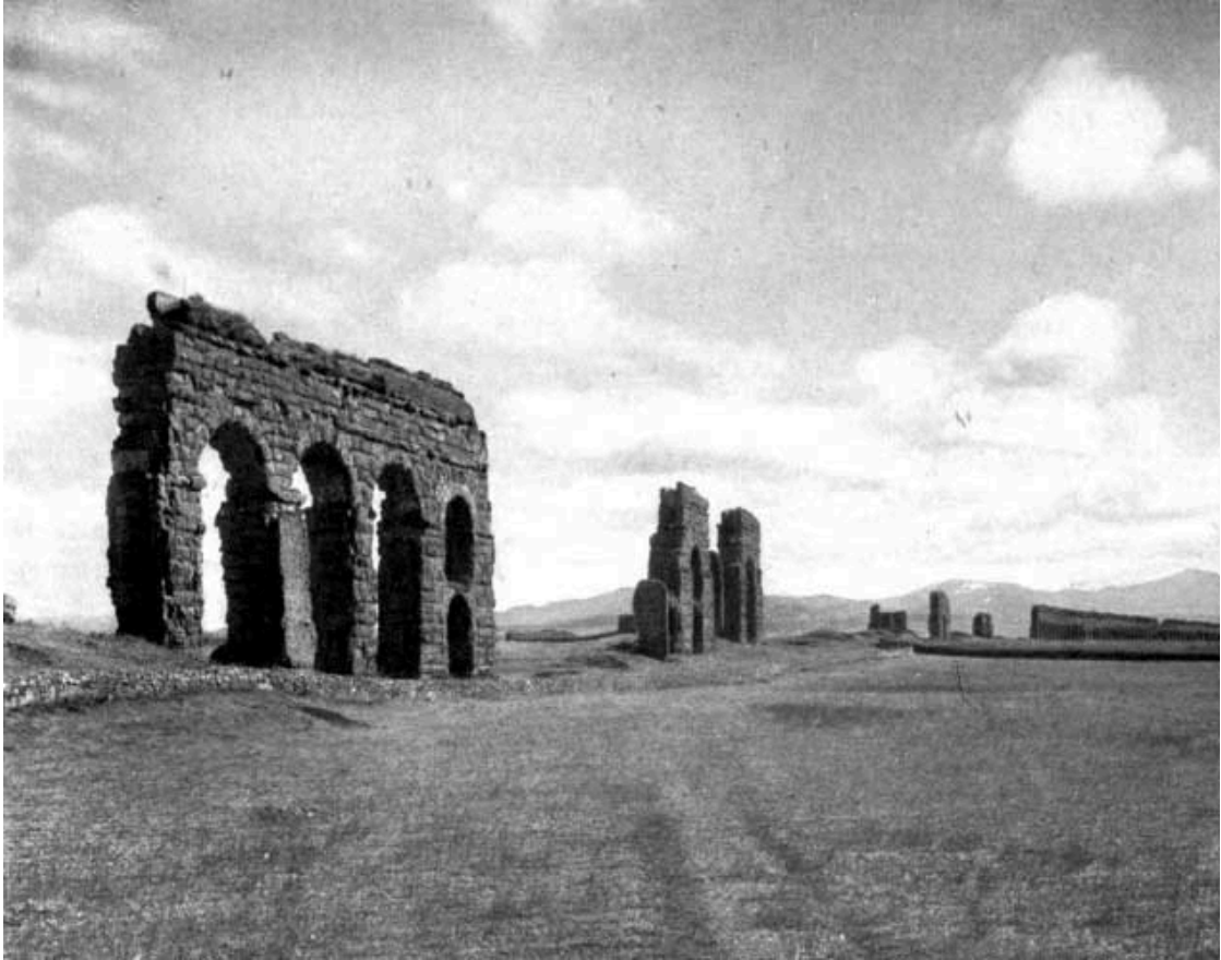
THE CAMPAGNA AND RUINS OF THE CLAUDIAN AQUEDUCTS, ROME.
