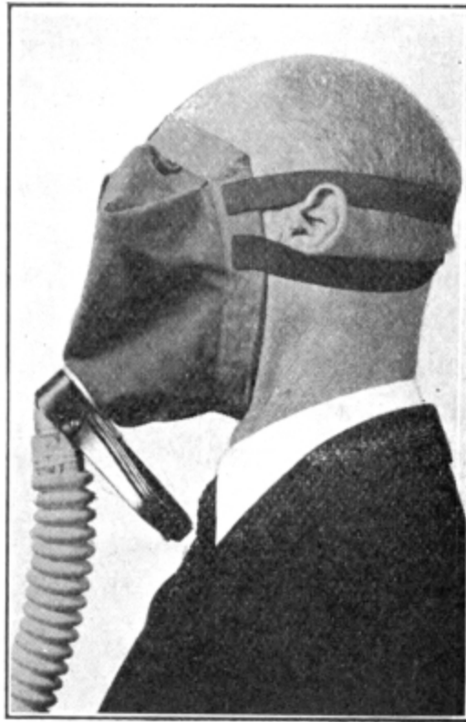
FIG. 44.—Early Type of Standard (British) Box Respirator (S. B. R.)
