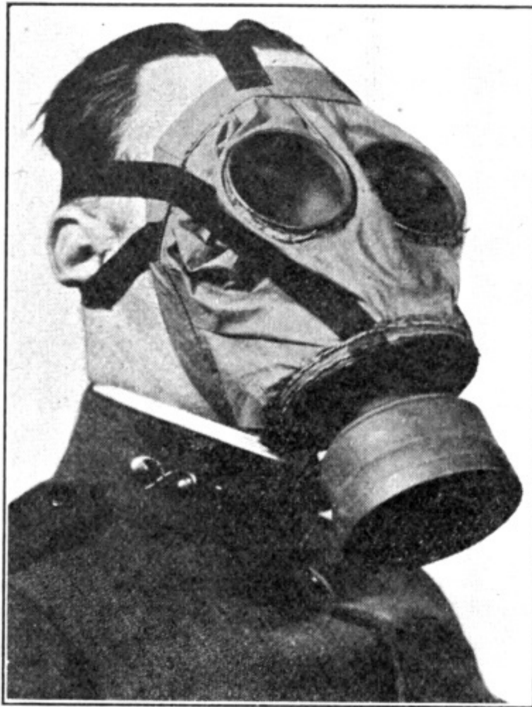
FIG. 64.—Early Type Navy Mask. Contains noseclip and mouthpiece.
