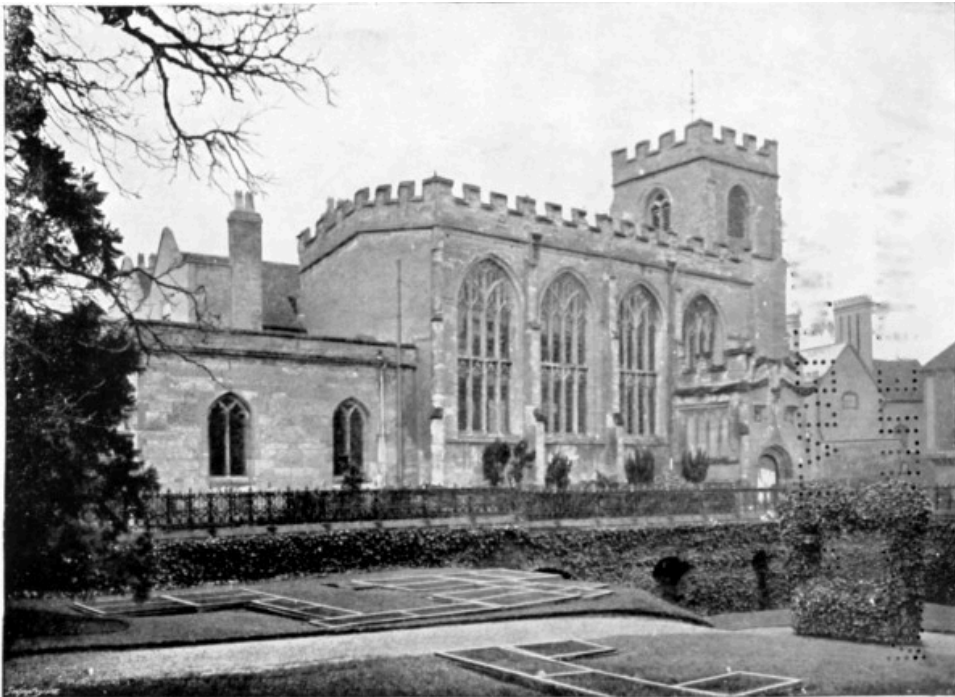
THE GUILD CHAPEL, FROM THE SITE OF NEW PLACE.
