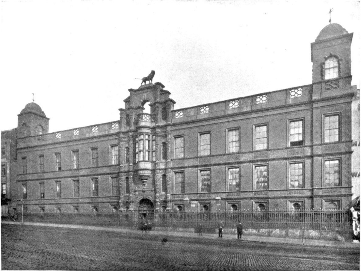
FIG. 79.—NORTH FRONT (BEFORE 1874).
