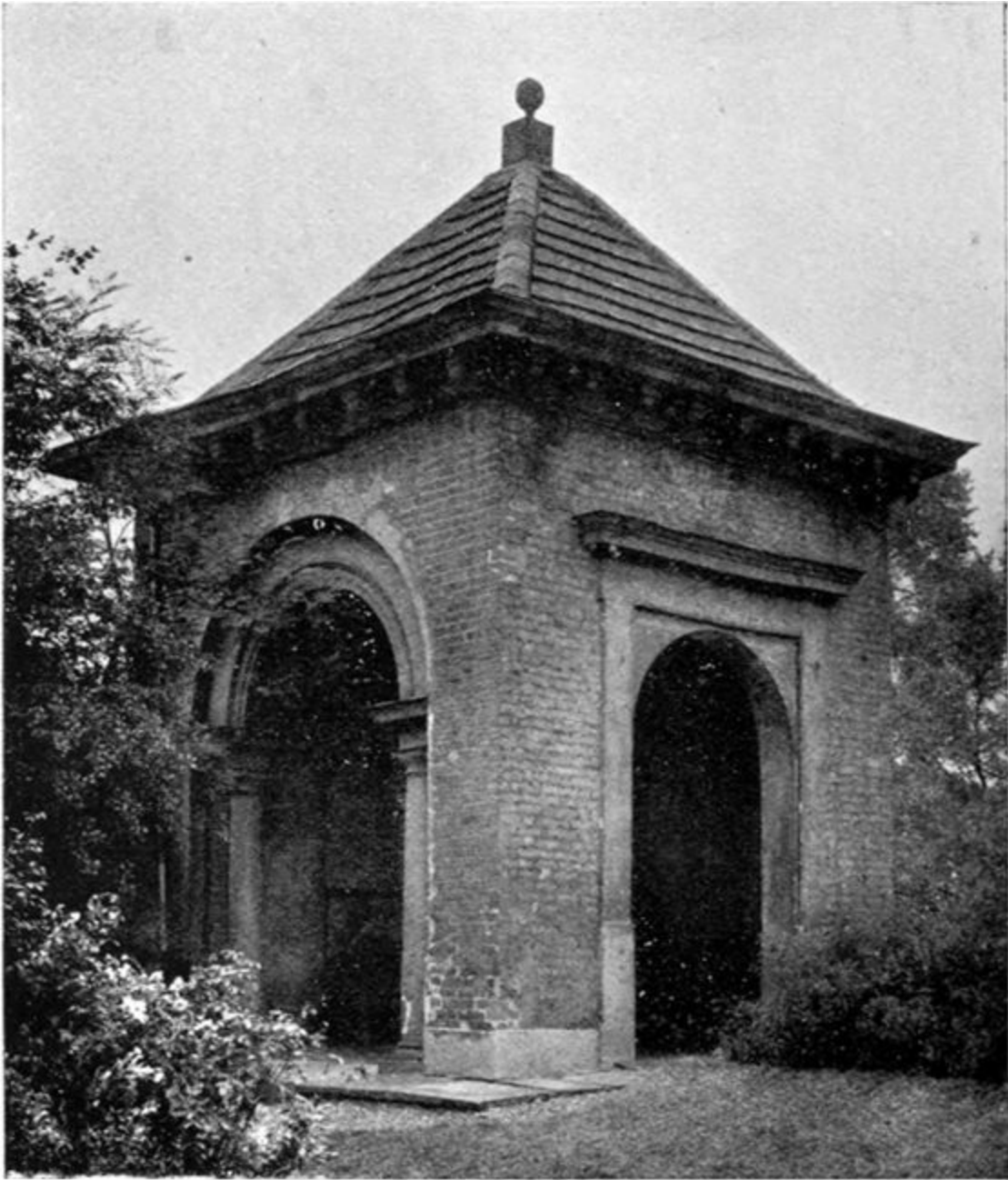
FIG. 161.—Garden House at Croom's Hill, Greenwich.
