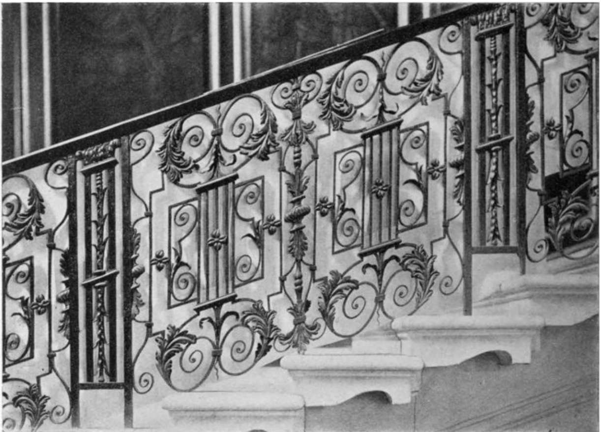
FIG. 264.—Balustrade to the King's Staircase, Hampton Court.
