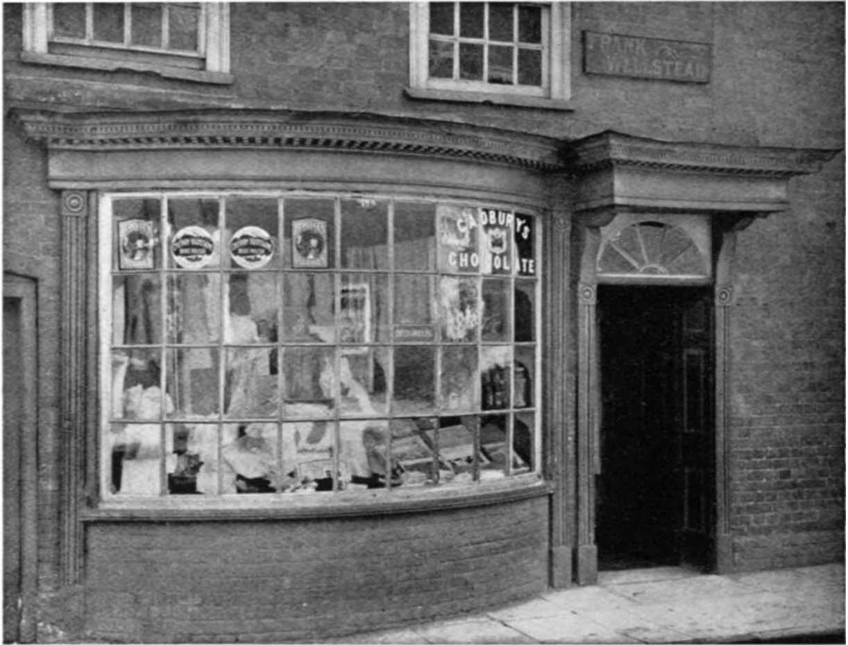
FIG. 218.—Shop in East Street, Wareham, Dorset.
