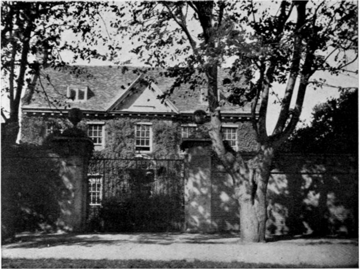
FIG. 206.—House at Ely, Cambridgeshire.
