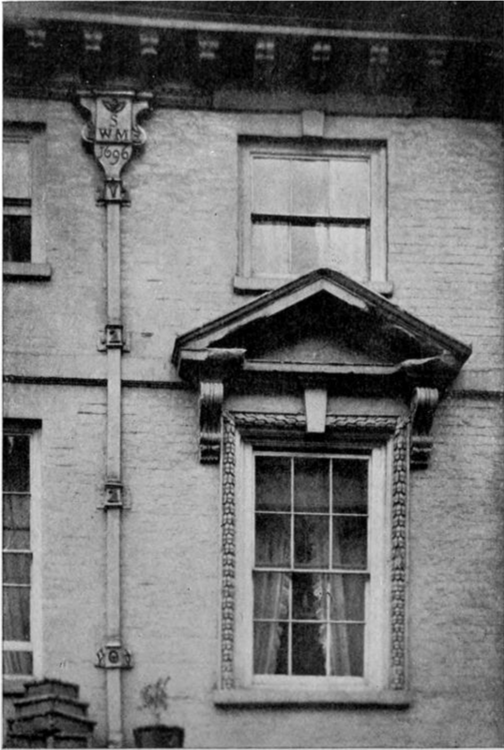
FIG. 273.—Lead Rain-Water Head at the Aylesford Hotel, Warwick.
