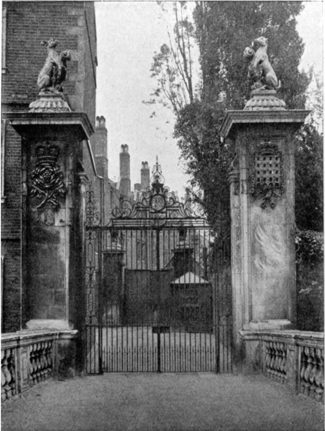
FIG. 243.—Gate-Piers at St John's College, Cambridge.
