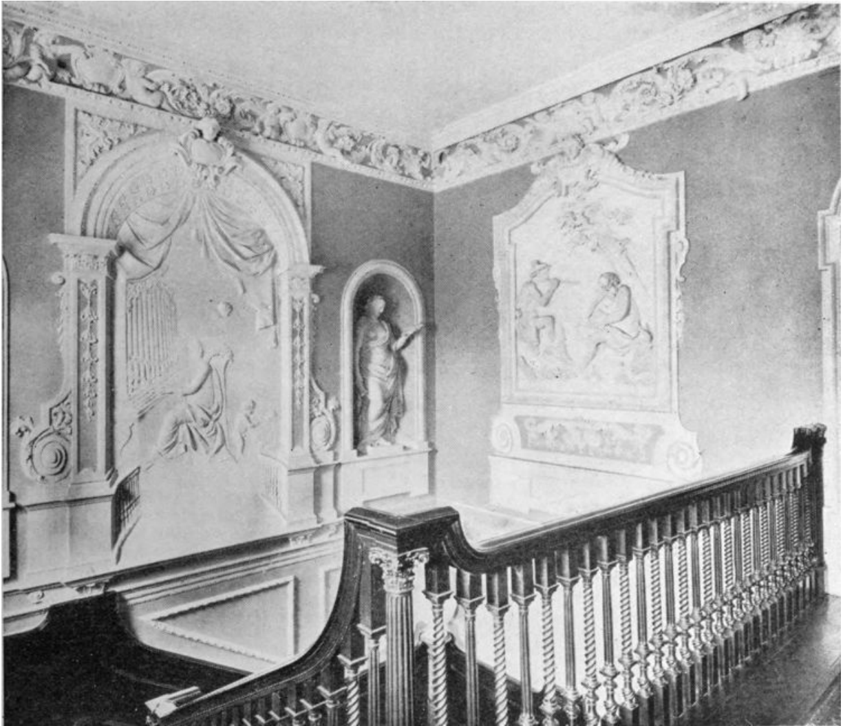
FIG. 289.—House in Queen Square, Bath.
