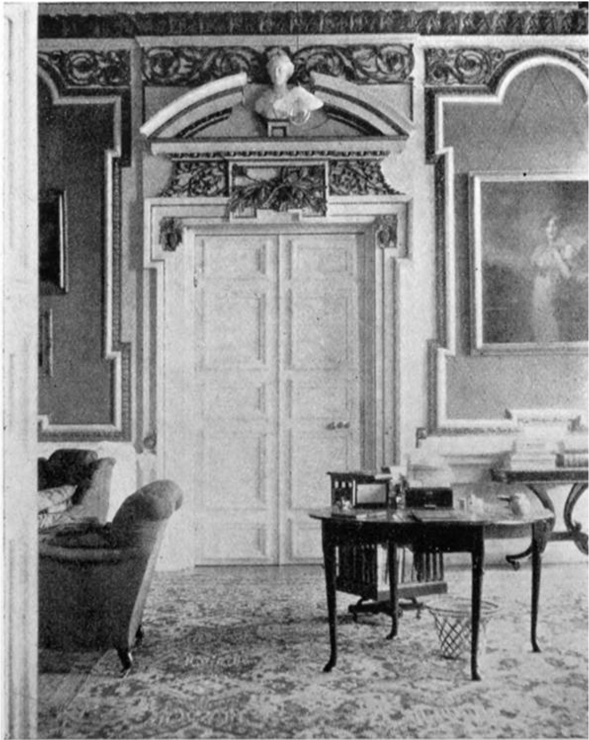
FIG. 129.—Stapleford Park, Leicestershire. Doorway in the Library.
