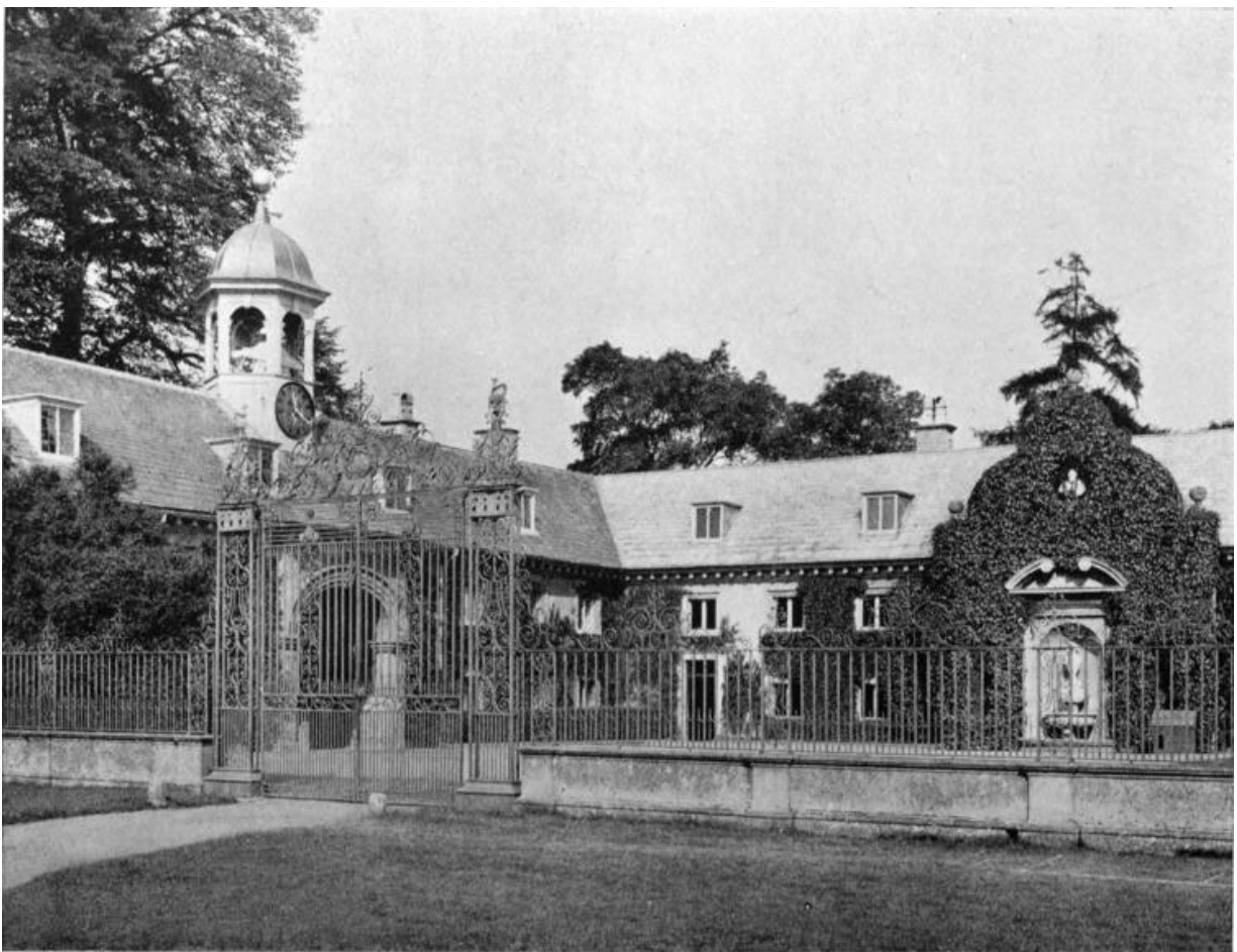
FIG. 106.—IRON SCREEN AND GATES, BELTON HOUSE.
