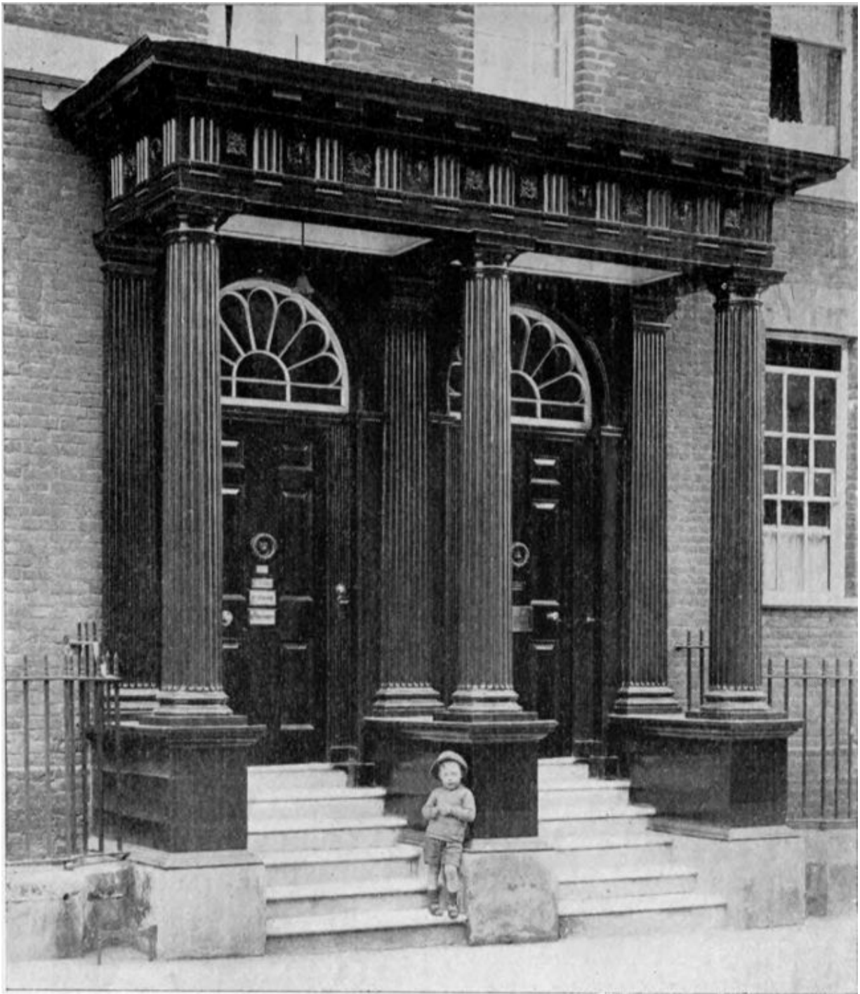
FIG. 256.—Doorways at Norwich.
