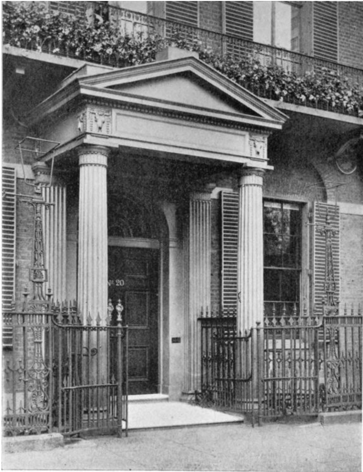
FIG. 197.—Entrance and Porch at 20 Portman Square, London.
