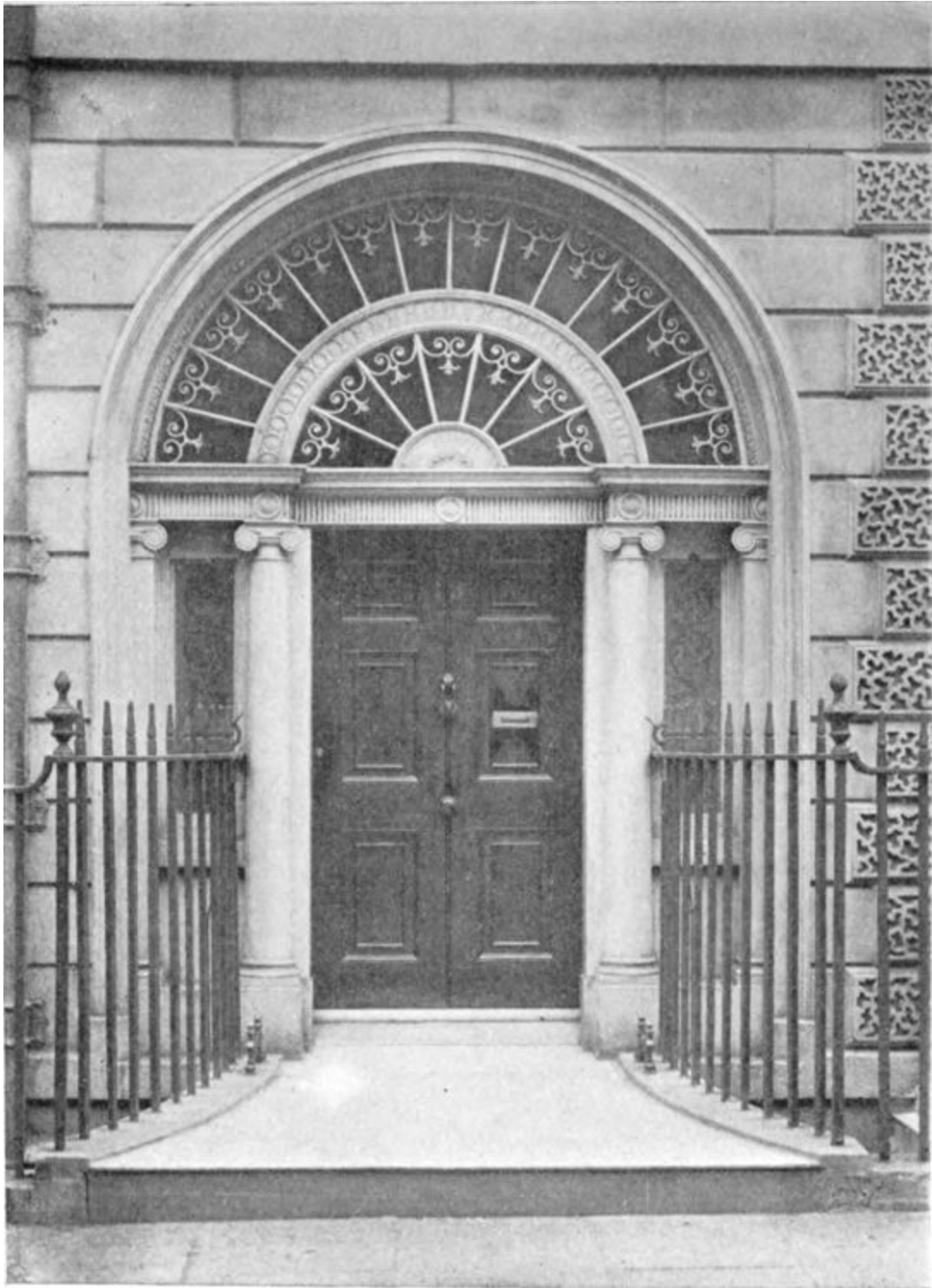
FIG. 196.—Doorway in Mansfield Street, London.
