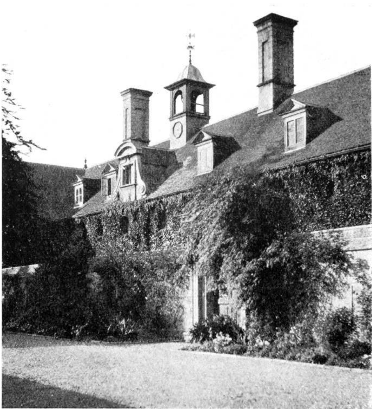
FIG. 51.—Thorpe Hall. The Stables.
