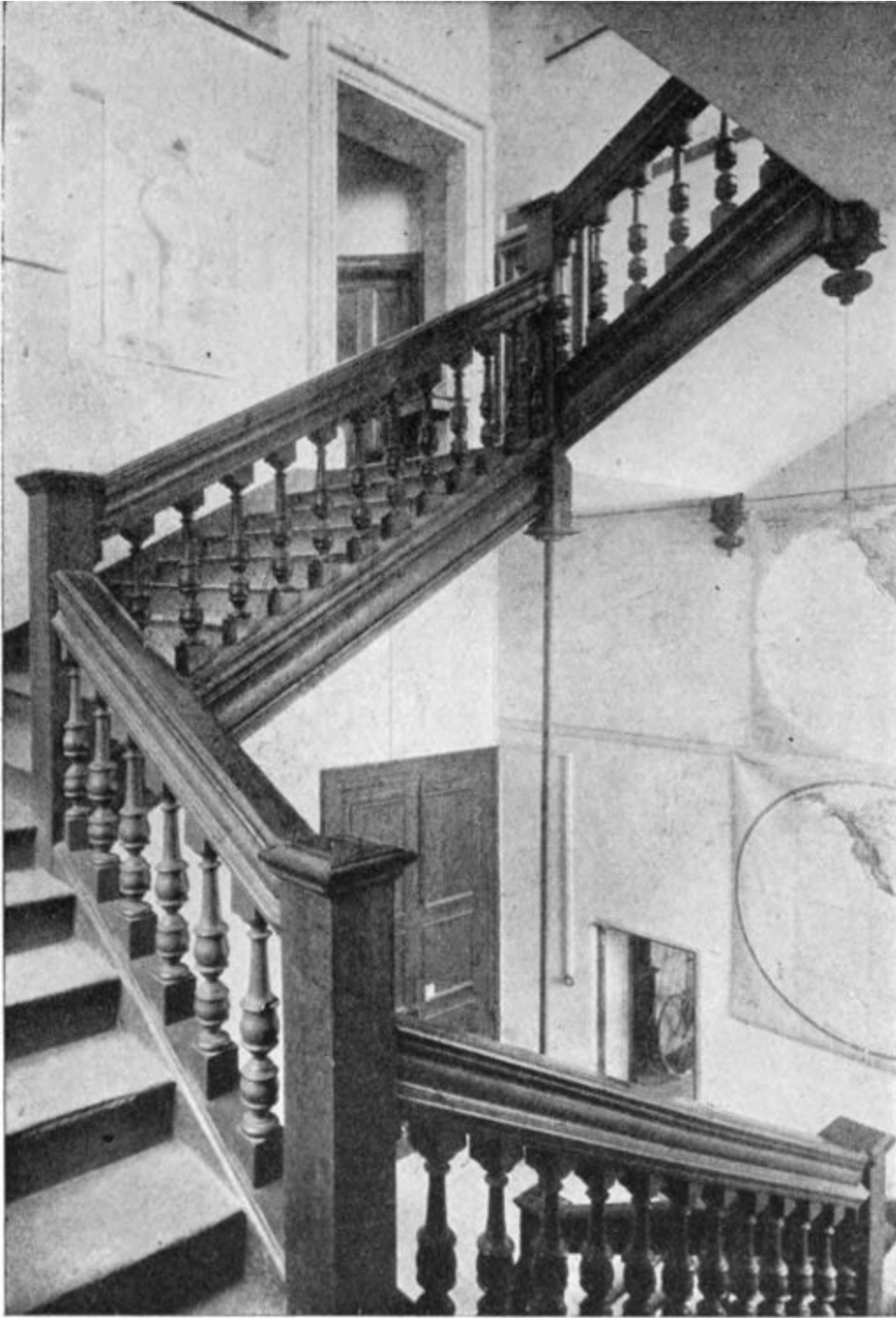
FIG. 277.—Staircase, Ashmolean, Oxford.
