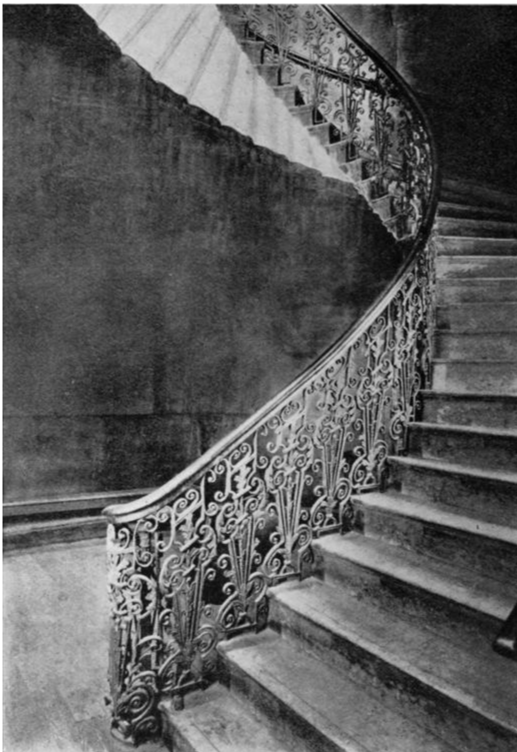
FIG. 281.—Staircase at No. 35 Lincoln's Inn Fields.
