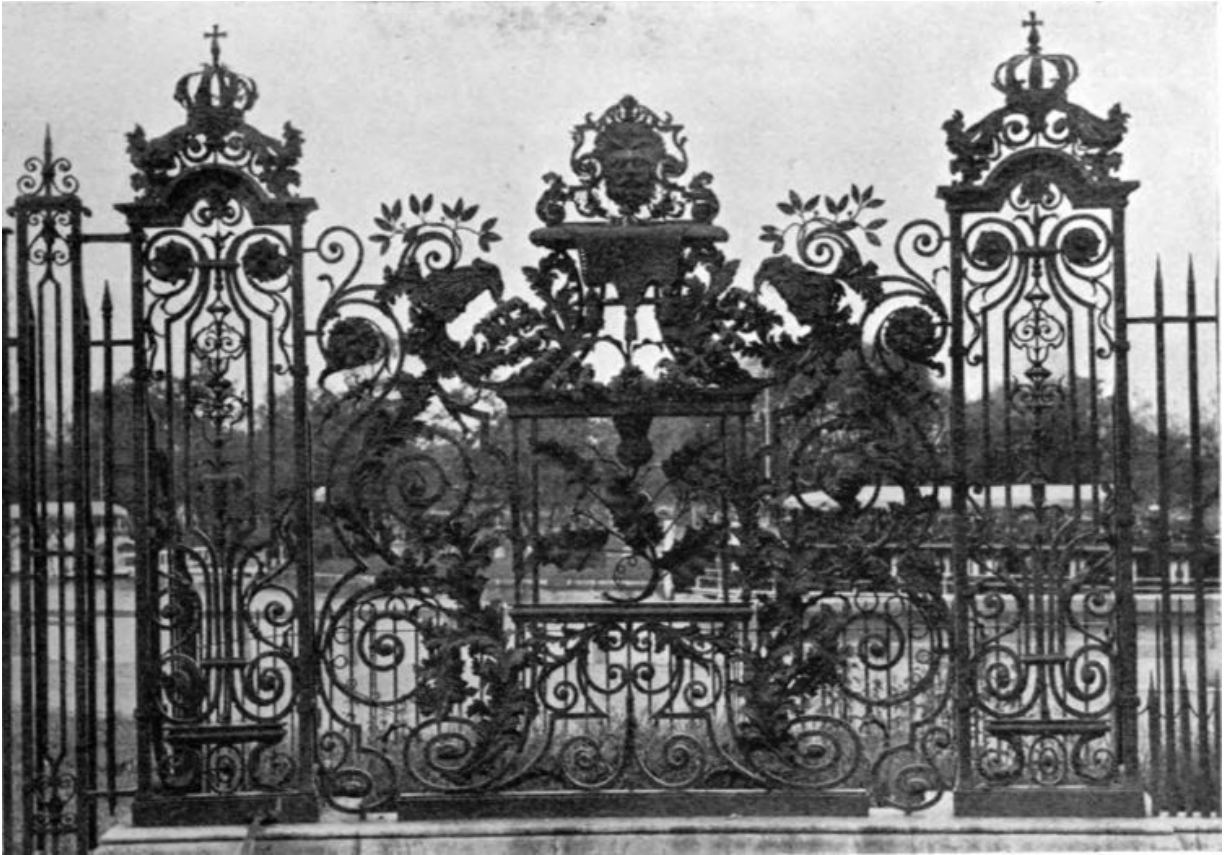
FIG. 262.—Part of Iron Screen, Hampton Court Palace.
