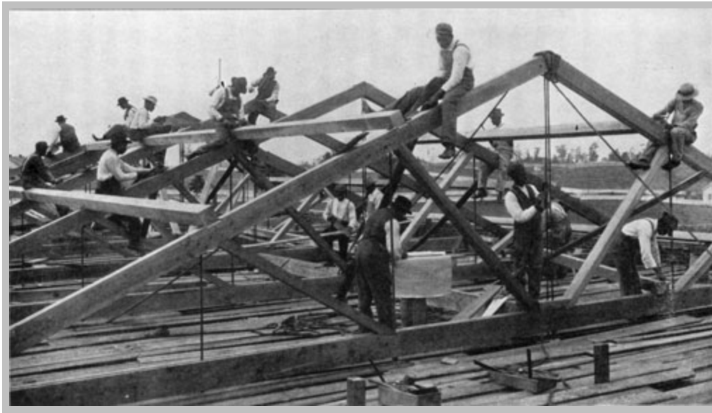
Tuskegee in the making. Nothing delighted Mr. Washington more than to see his students doing the actual work of erecting the Tuskegee Institute buildings. A group of students raising the roof on one of the buildings.
