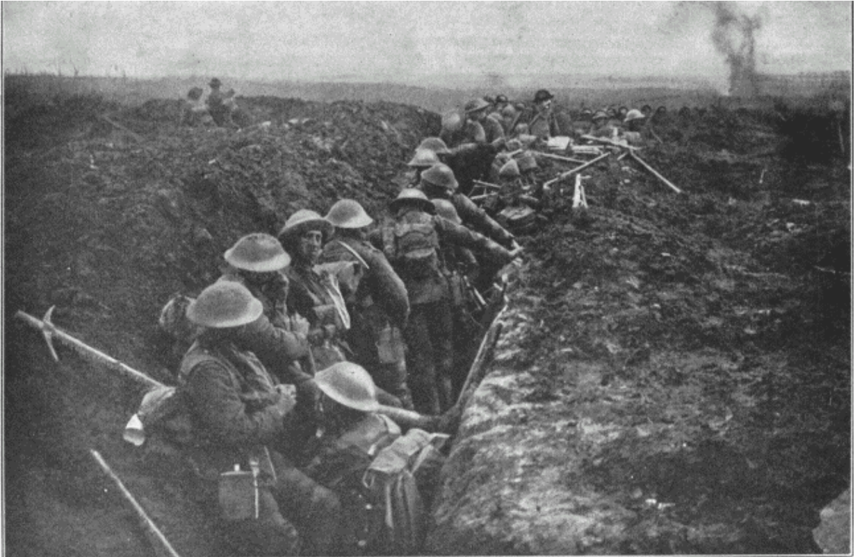
In the supports, waiting to advance
