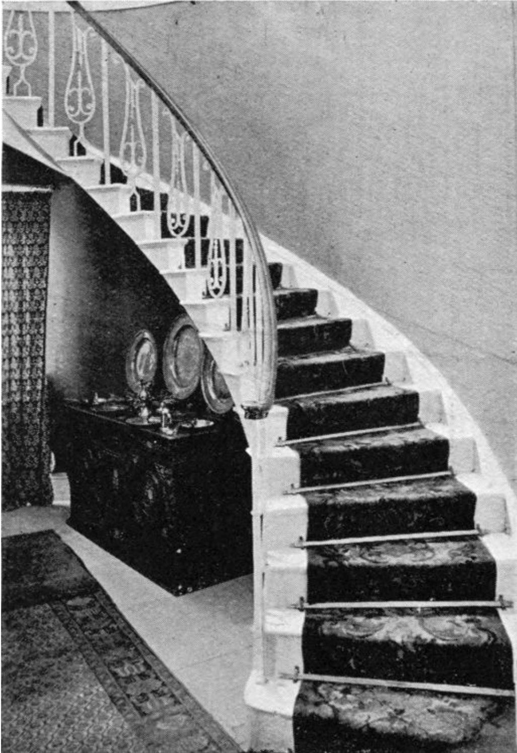
214. Staircase in Badow House, Essex.
