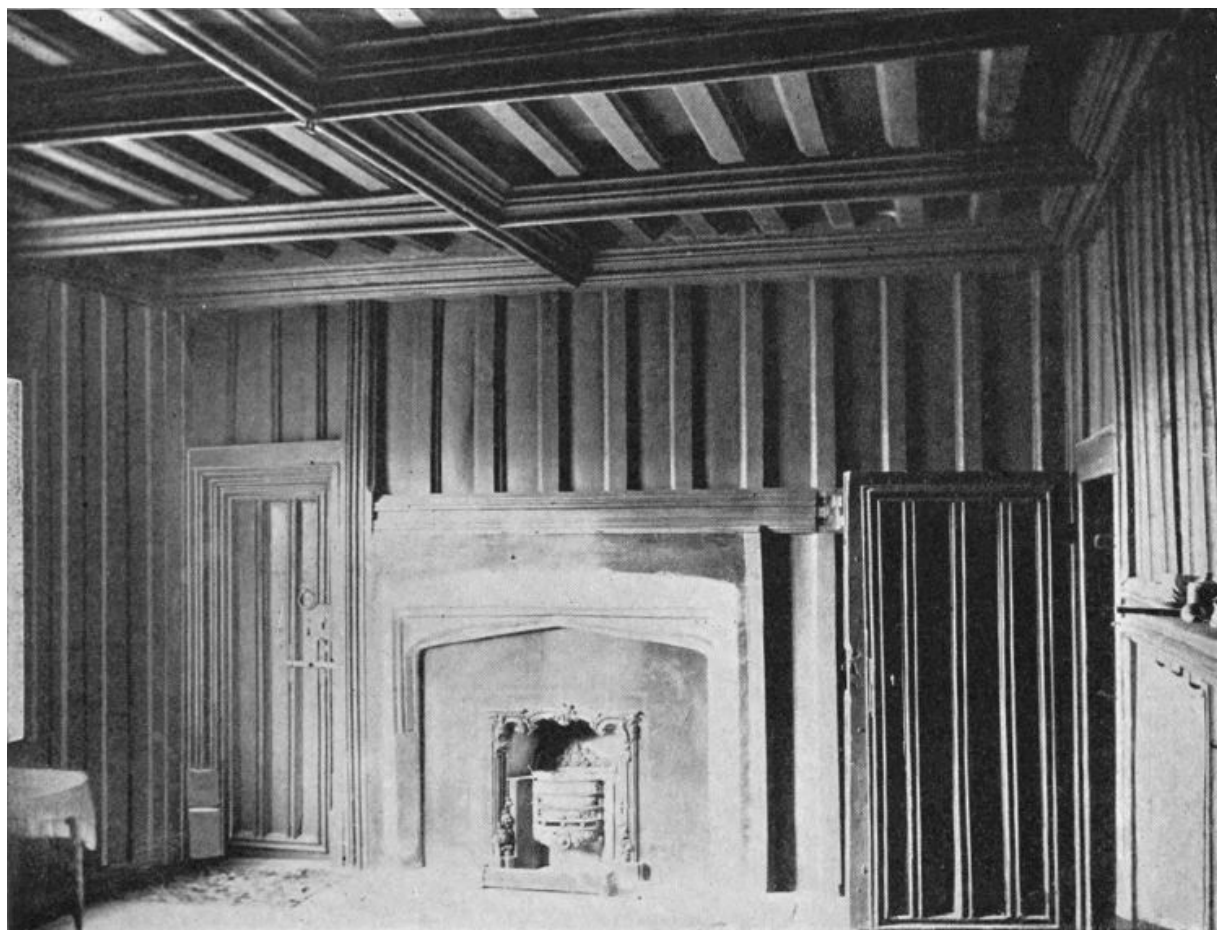
87. Crowhurst Place, Surrey. Ceiling with Moulded Beams.
