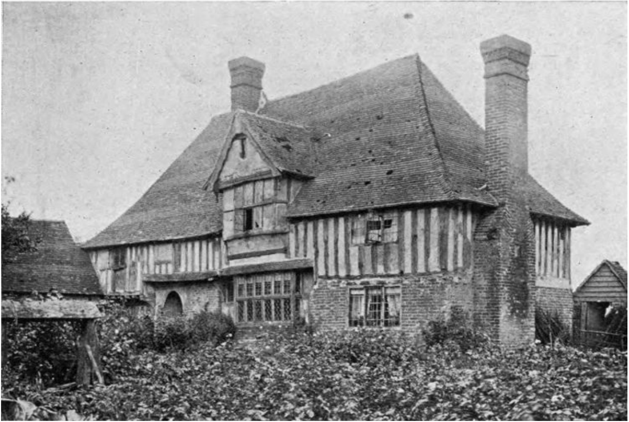
123. House at Brad Street, Kent.
