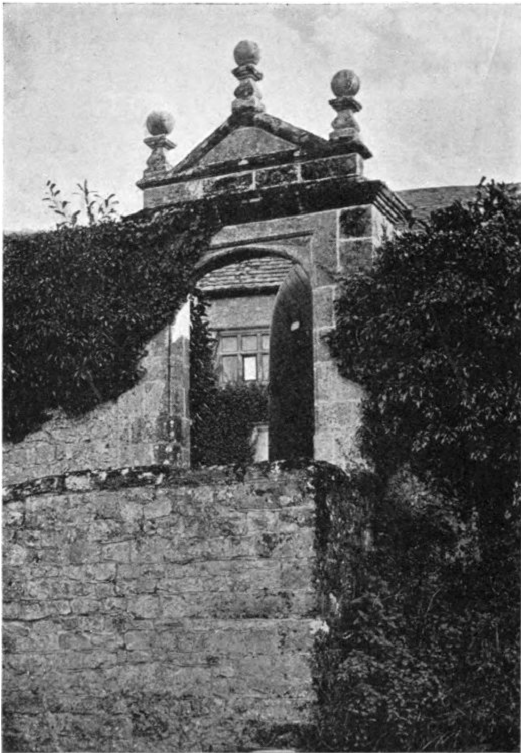
127. Entrance Gateway at West Burton, Sussex.
