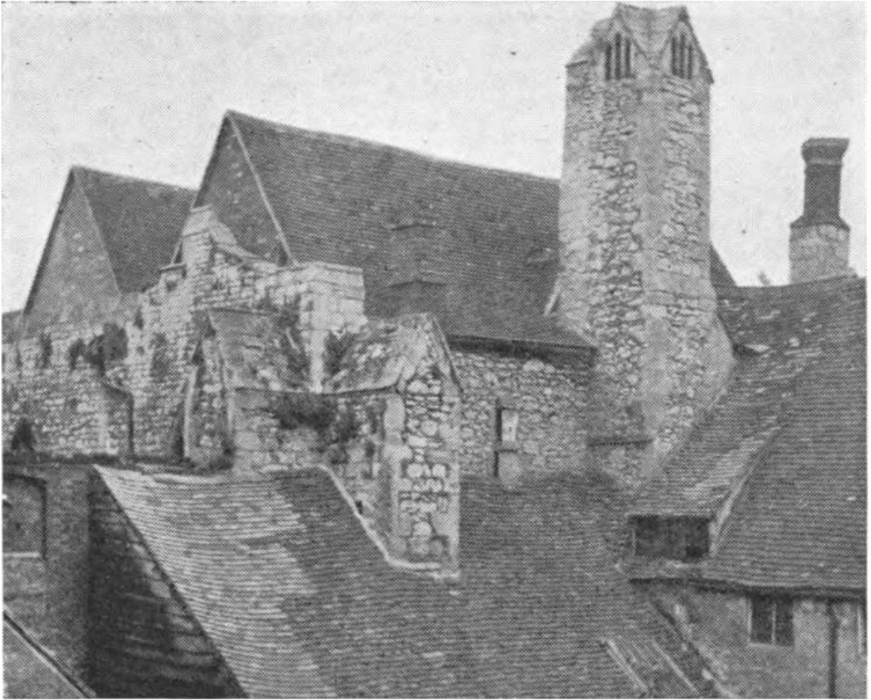
72. Abingdon Abbey, Berkshire. Chimney-shaft and Chimney-vent (13th cent.).
