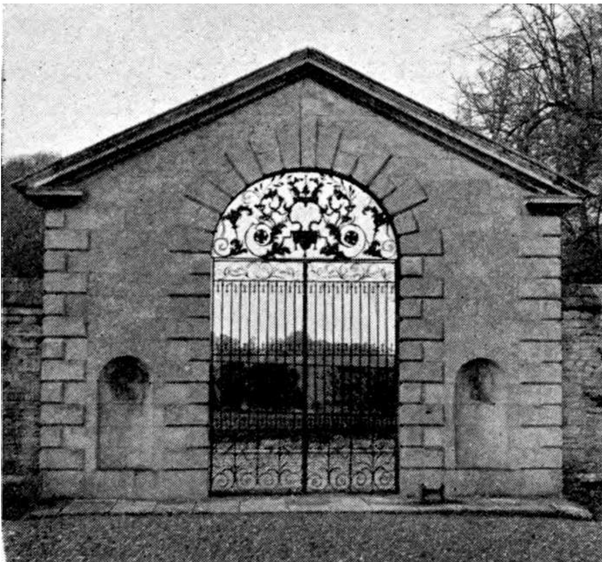
176. Drayton House, Northamptonshire. Gates in the Side of Fore-court ( cir. 1700).
