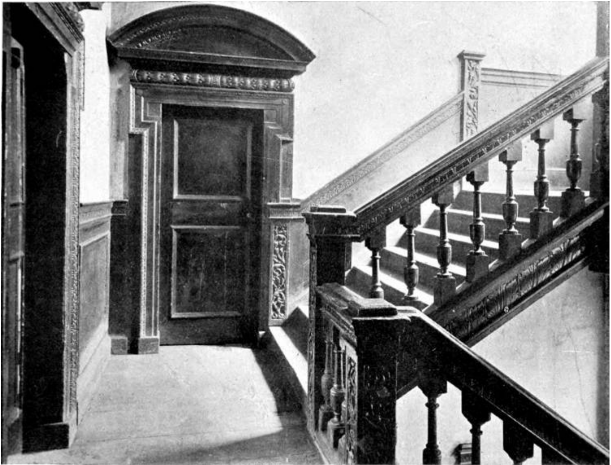
210. Staircase in a House in Love Lane, London (now destroyed). (Late 17th cent.)
