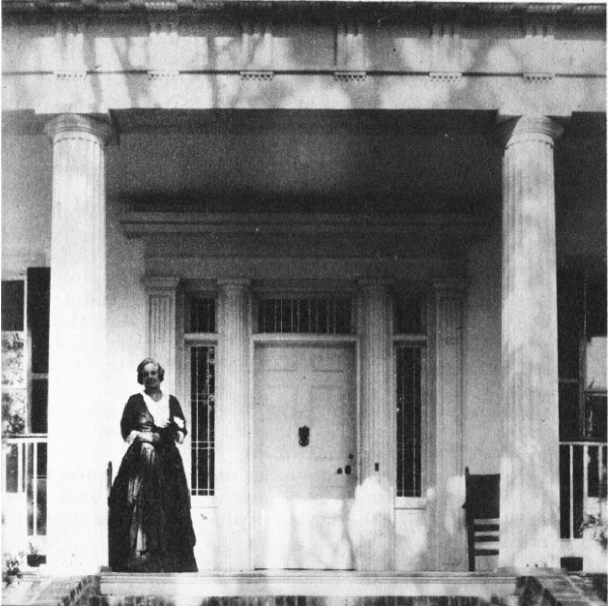
AN INTERESTING TREATMENT OF TRANSOM AND SIDE LIGHTS
