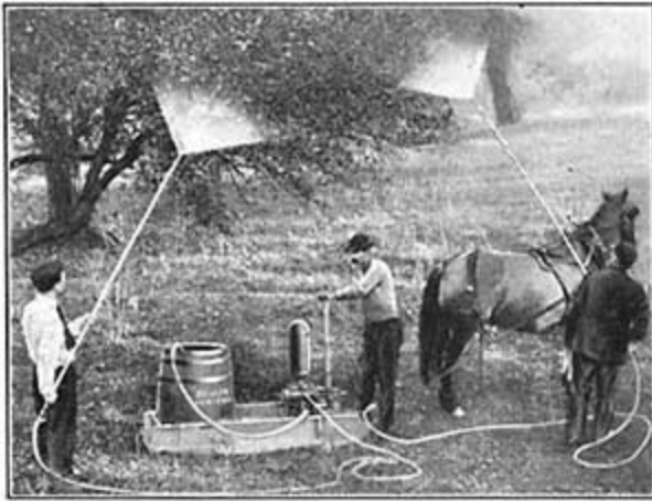
FIG. 143.—Spraying trees by means of a compression pump.
